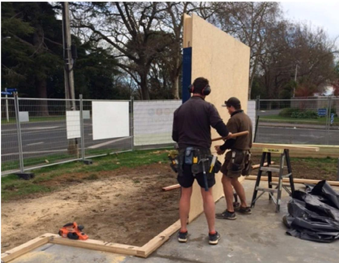
*Erecting structural insulated panels*
