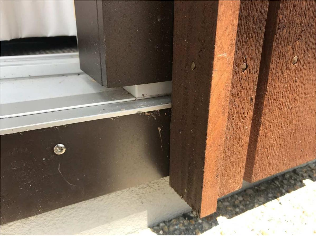
*Close up photo of lift and slide sill and jamb.*
