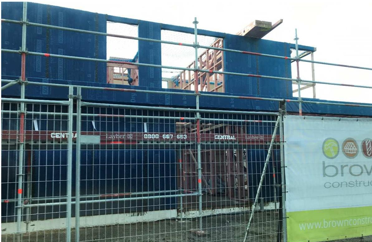
*Trusses stacked on top of erected walls prior to installation*
