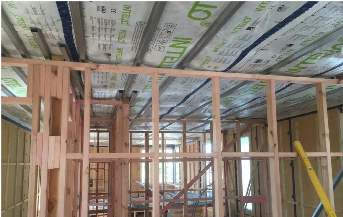
*Underside of roof showing Intello airtightness membrane*
