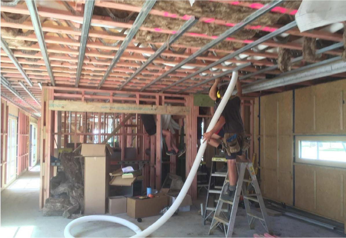
Construction photos showing installation of ducting within Posi Struts
