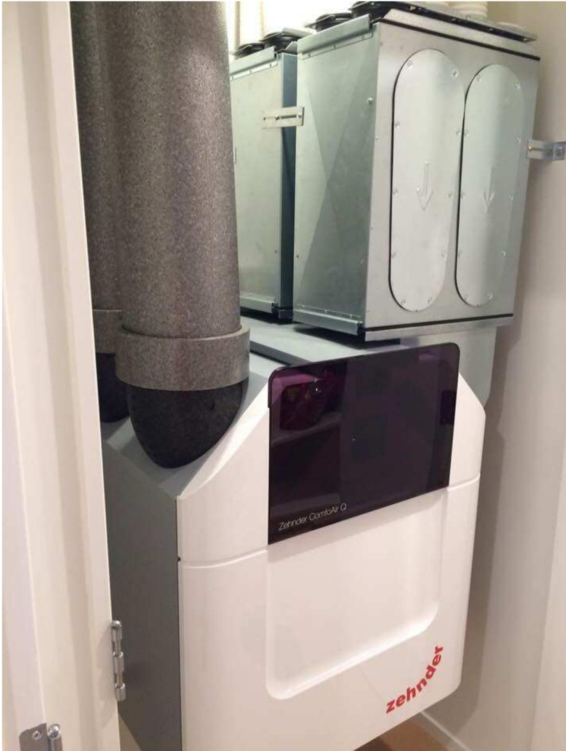
*Zehnder Comfoair Q350 with external supply and return to left and silencers/manifolds to the right separating to each room.*
