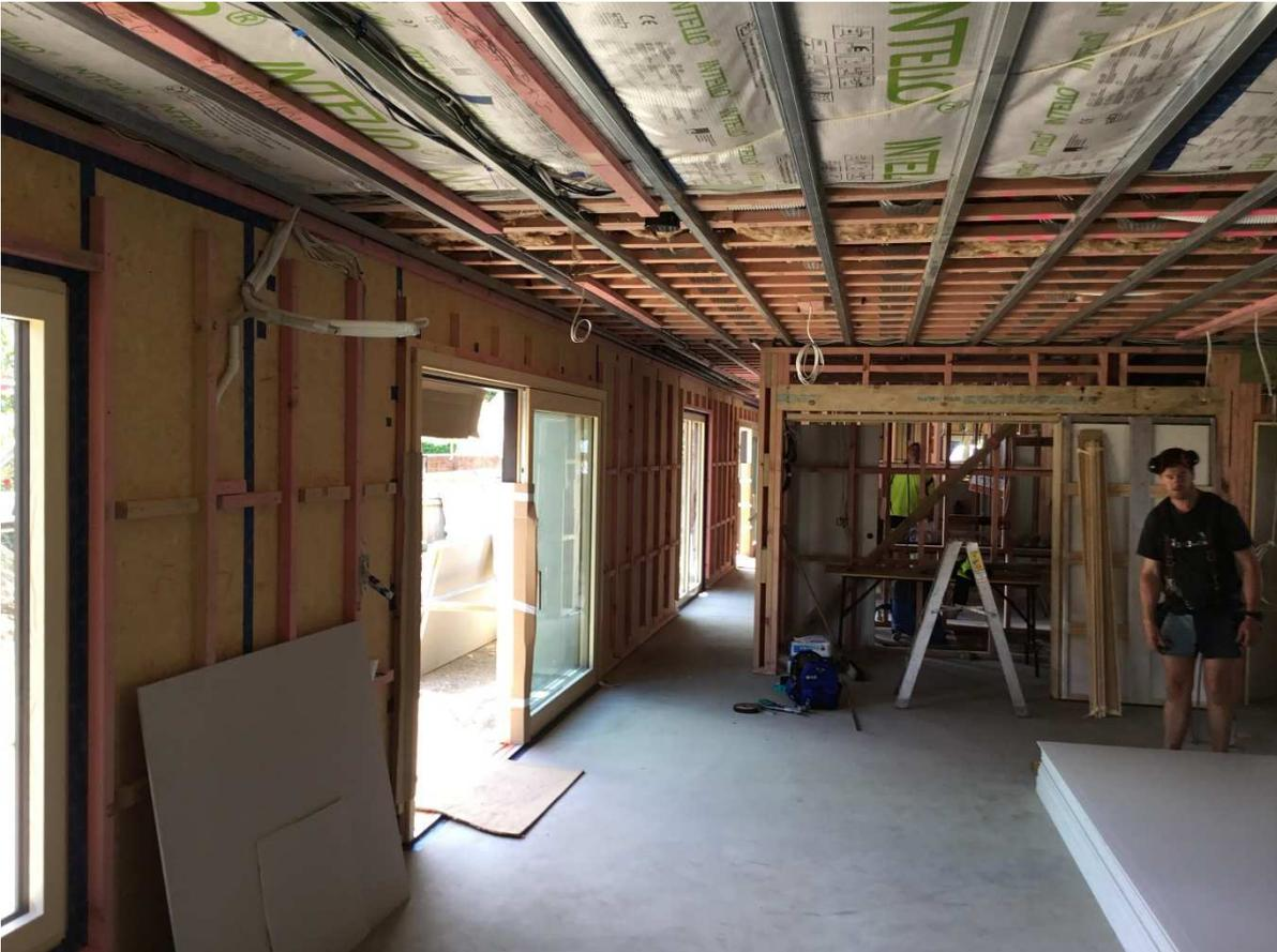
*Construction photo showing Proclima Intello airtightness membrane under lower roof section and wall panels taped using Teson Vana airtightness tape.*
