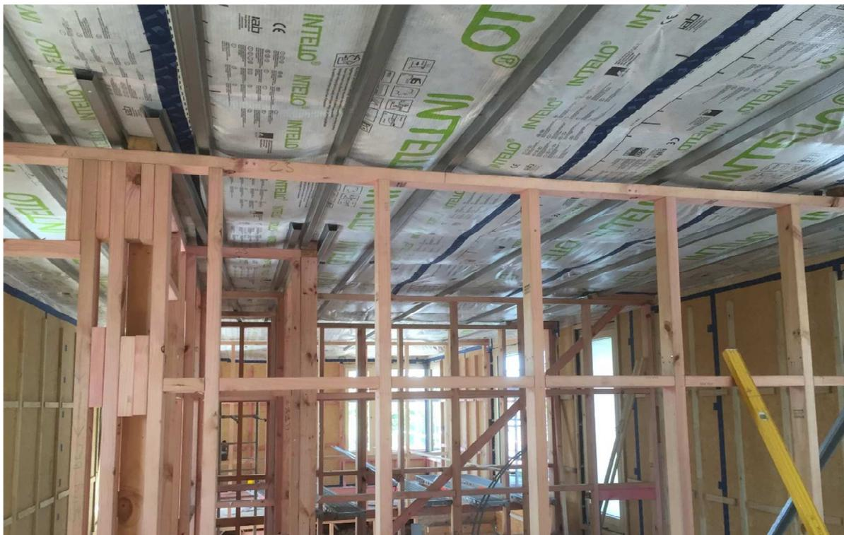
*Underside of roof showing Intello airtightness membrane*
