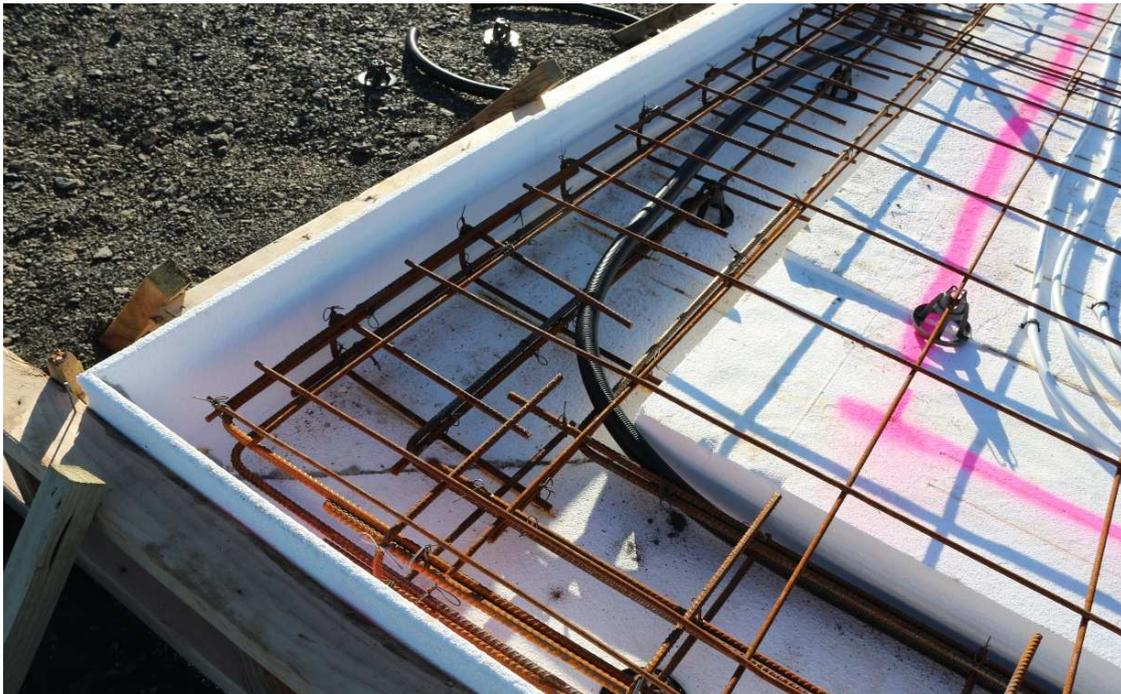
*Edge Foundation Detail. This photo is of a similar project except that in this phot the edge insulation is only 15mm thick rather than 30mm thick as it was in this project.*
