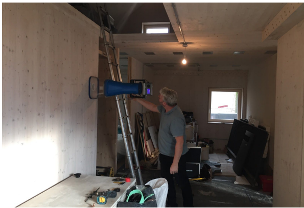
Construction photos of the duct install and terminal commissioning and a photo of the MVHR unit in place.
