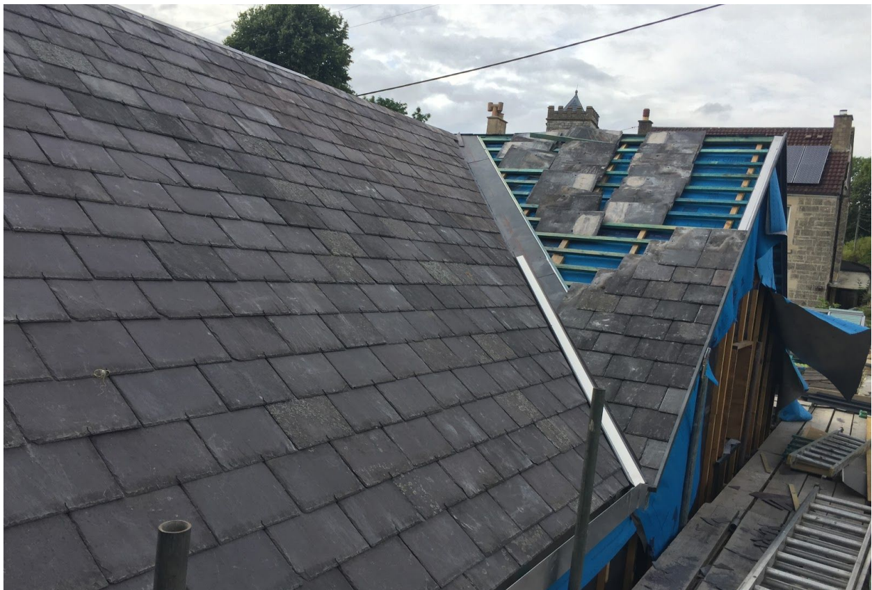
Construction photo nearing completion of the roof, showing reclaimed slates and concealed gutter
