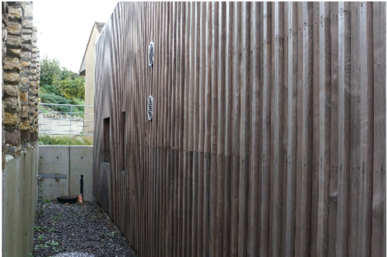
North. Rear elevation with minimal glazing. MVHR intake & exhaust terminals visible.
