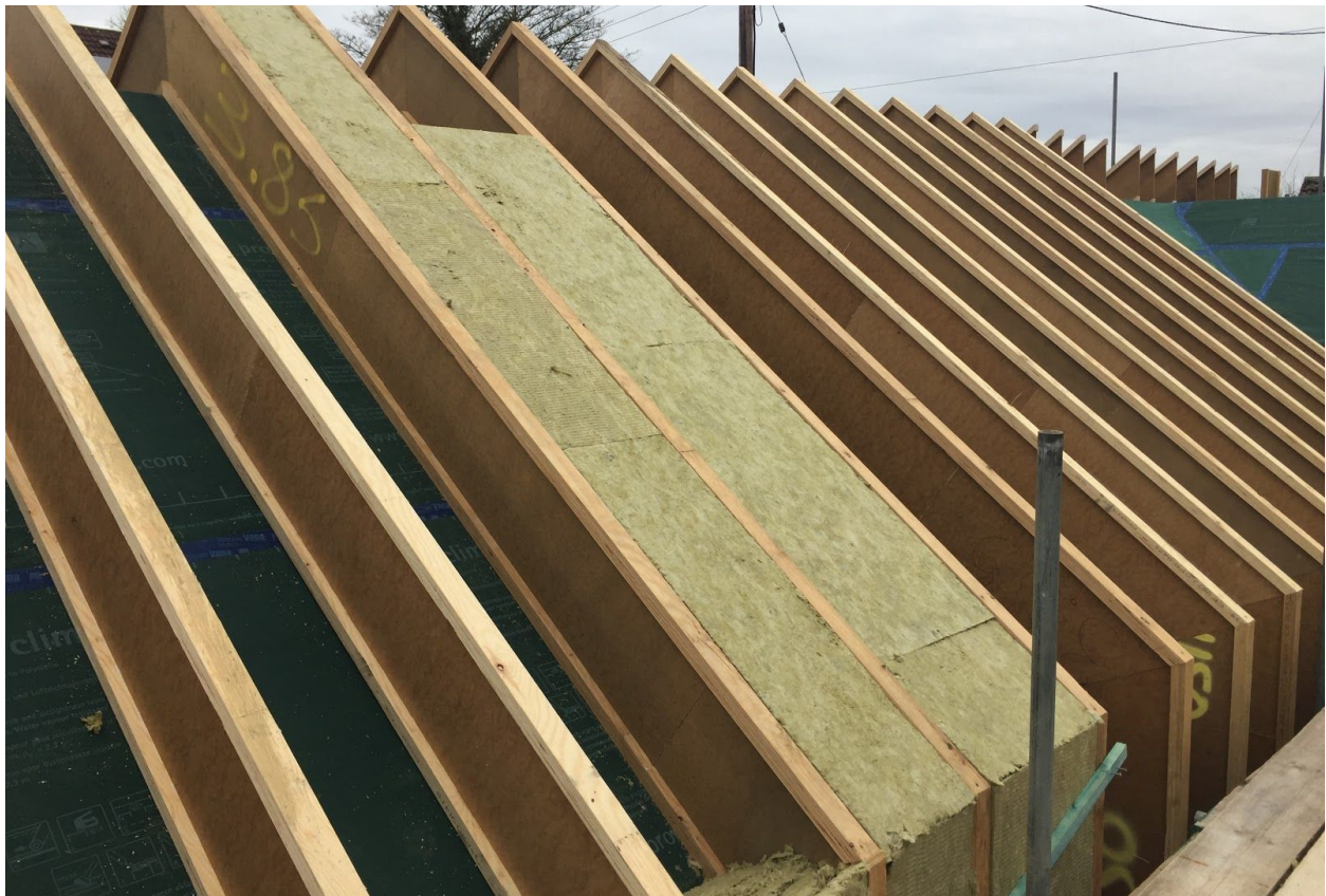
Construction photo showing the 'Larsen Trusses' with mineral wool infill.
