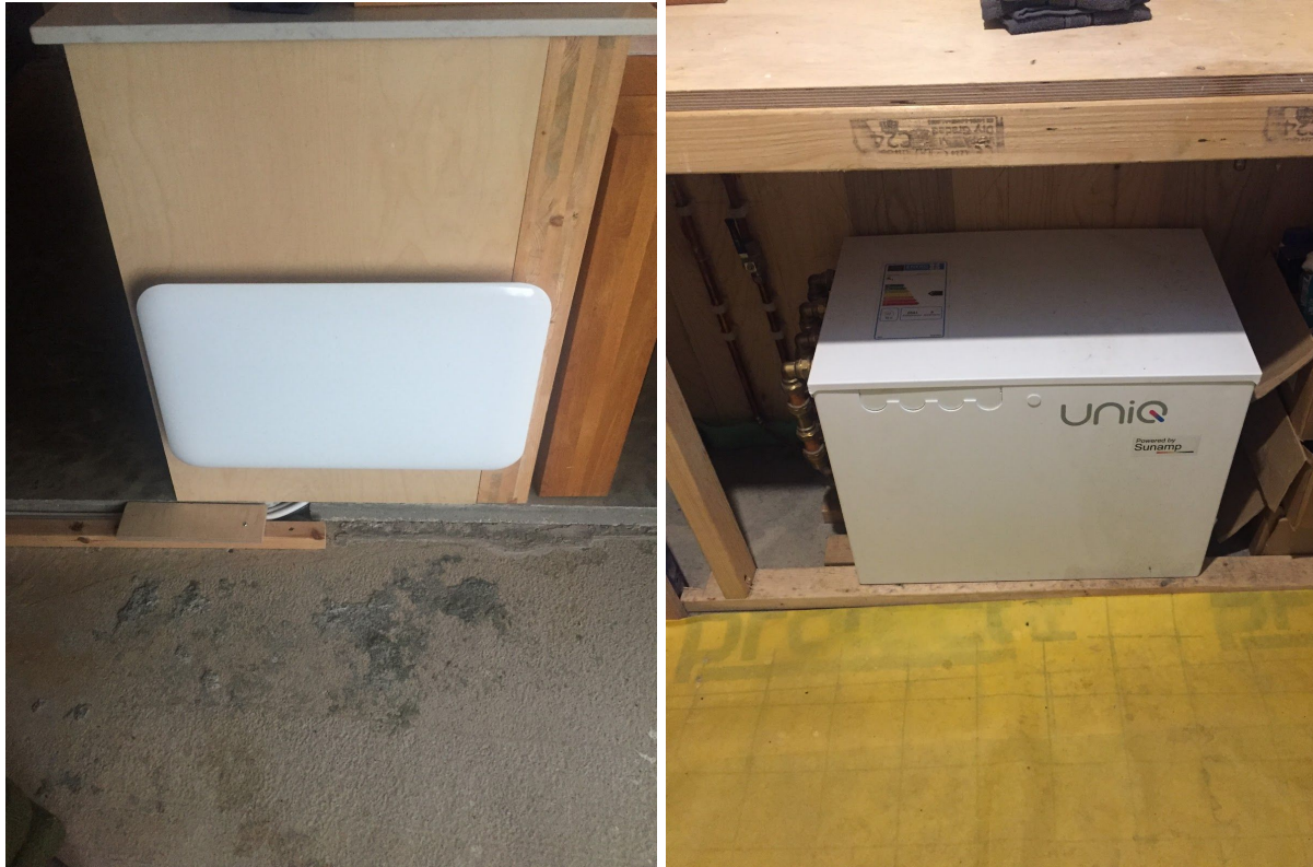
Construction photo of a panel heater (living space) and heat battery (en-suite) installed.
