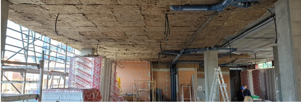
First Floor under and top insulation installation (Source: RLA)
