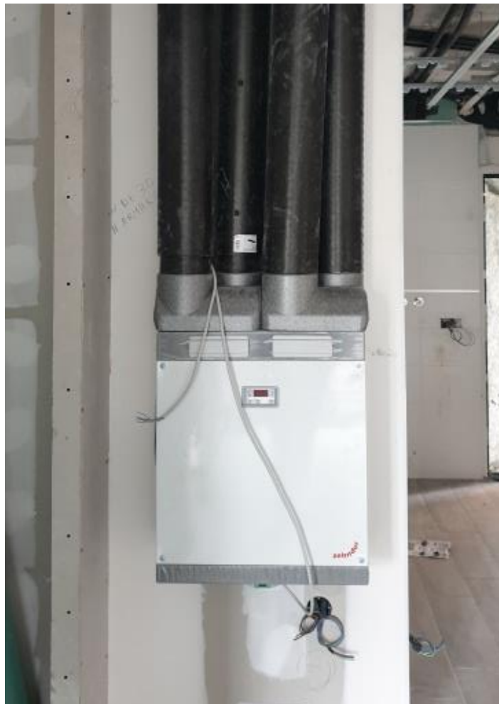
Ventilation unit (Source: RLA)
