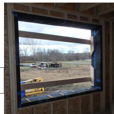
Insulation wrapped with Air Barrier
