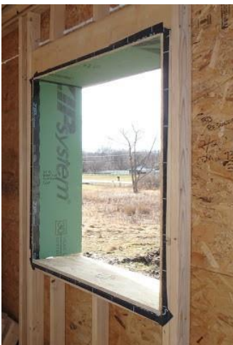
Bucks were built with the window sheathing cutouts
