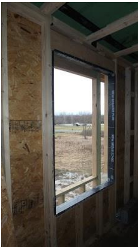
Air Barrier brought to inside
