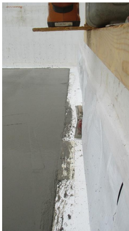
Slab Poured to Perimeter EPS
