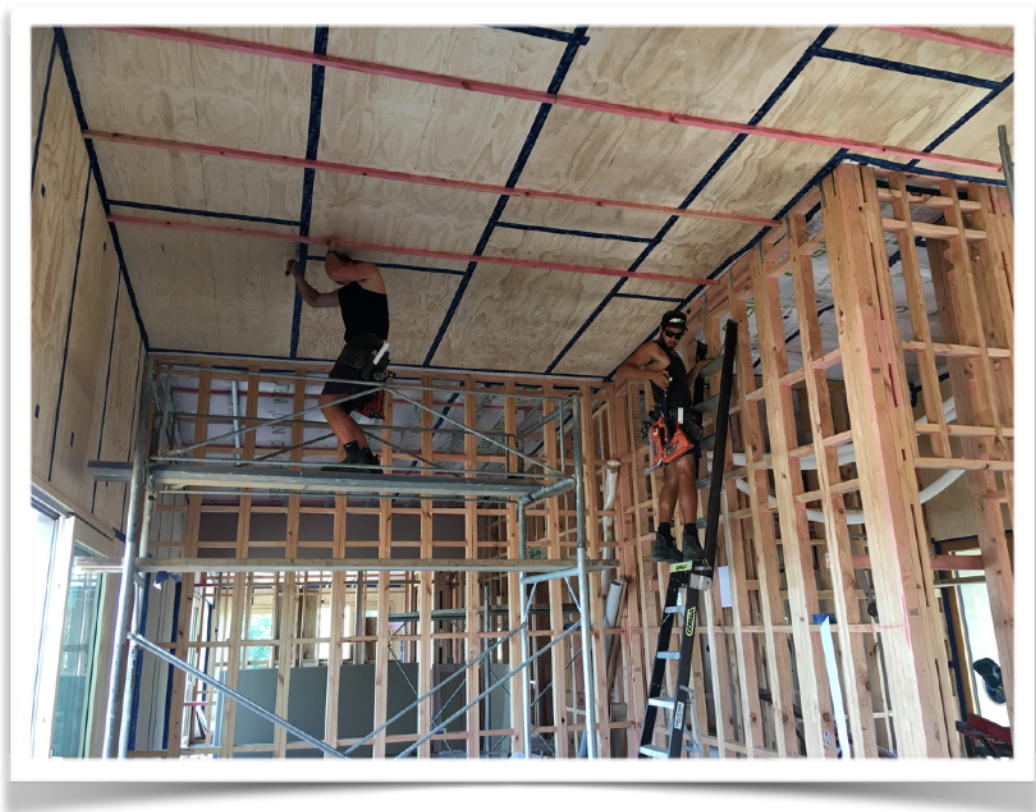
Ply airtightness on ceiling
