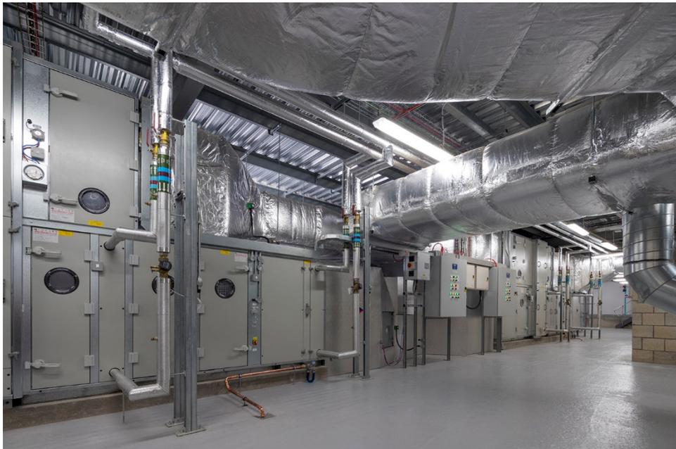
AHU installation in basement plantroom
