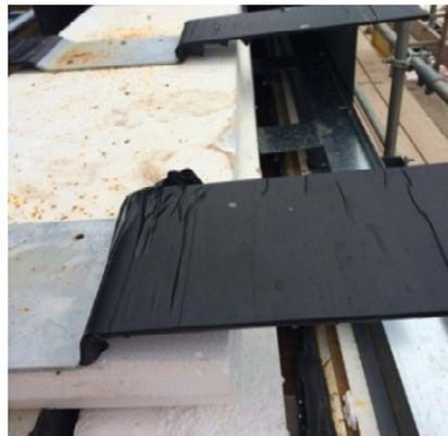
Images showing installation of continuous insulation on roof/wall parapet
