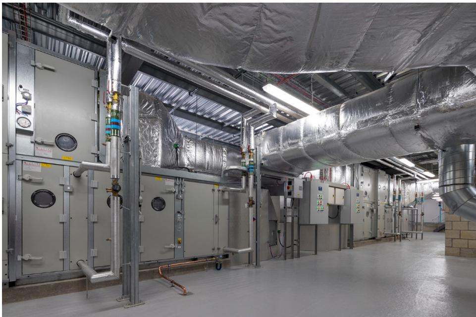
AHU installation in basement plantroom
