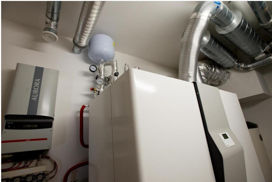
The air intake of the LWZ 304 ventilation unit is connected to the rehau AWADUKT THERMO air-to-ground heat exchanger which exploits the energy storage capacity of the soil to meet the heating and cooling needs inside the houses is the first exchanger with pipes equipped with an internal antimicrobial layer, which guarantees healthy fresh air, improving living comfort and energy
