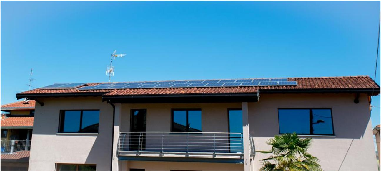
The photovoltaic system makes the house self-sufficient on the side of electricity production, with a self-consumption rate of approximately 26.2%.
