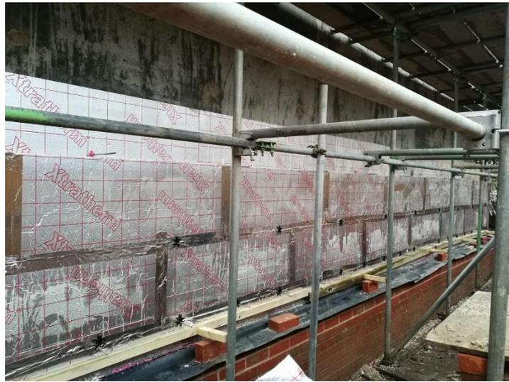
**Wall to wall junction- gaps between boards will filled with low-expansion foam:**
