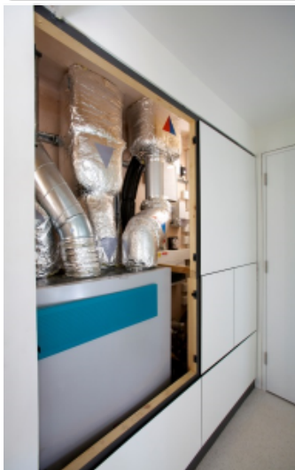
Schematic Diagram of MVHR unit (above left) and as Installed (above right)
