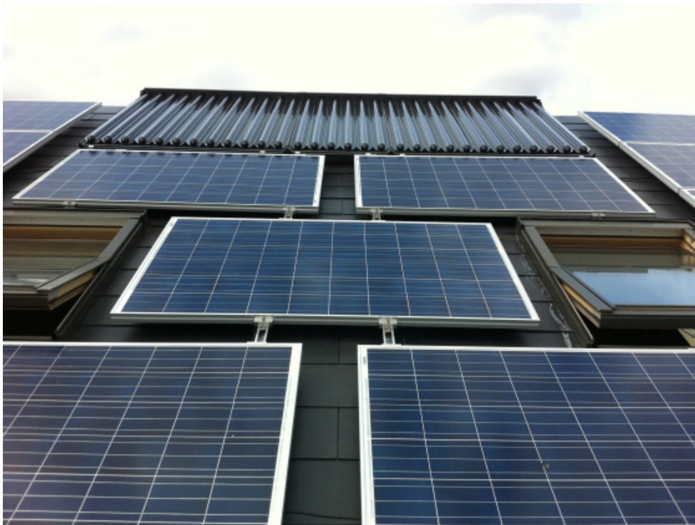
Solar Photo-voltaic Panels and Solar Thermal Evacuated Tubes
