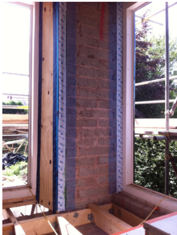
Air-tightness Certificate (above left) and Diligent Window/Wall Junction Installation (above right)
