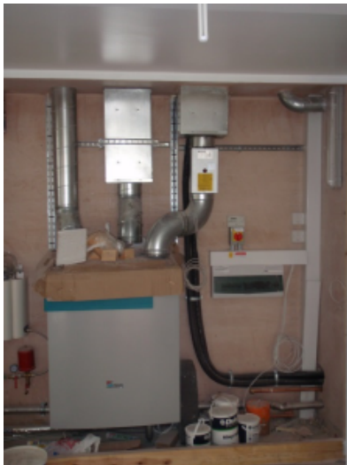
First Fix of MVHR Ductwork in Service Riser
