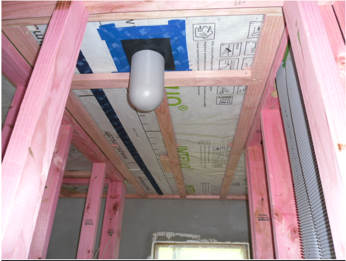
Ventilation ducts installed in the first floor ceiling
