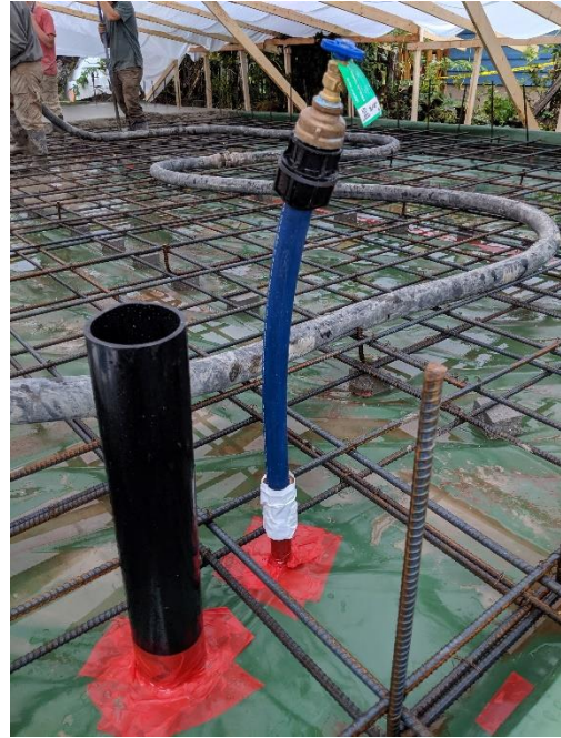
Slab rebar and building services penetrations
