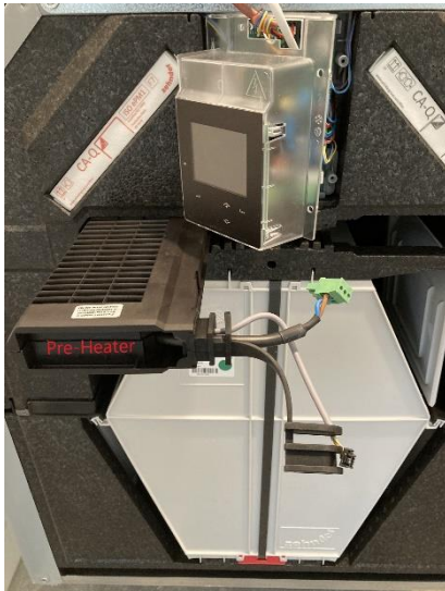
HRV built-in pre-heater unit
