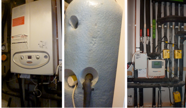
Fig 21 showing modulating boiler 100mm insulated cylinder and insulated pipework
