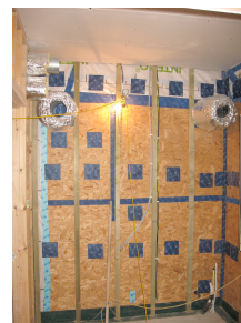
Fig 13 sealing with Proclima tape where Cellulose was blown into stud wall.
