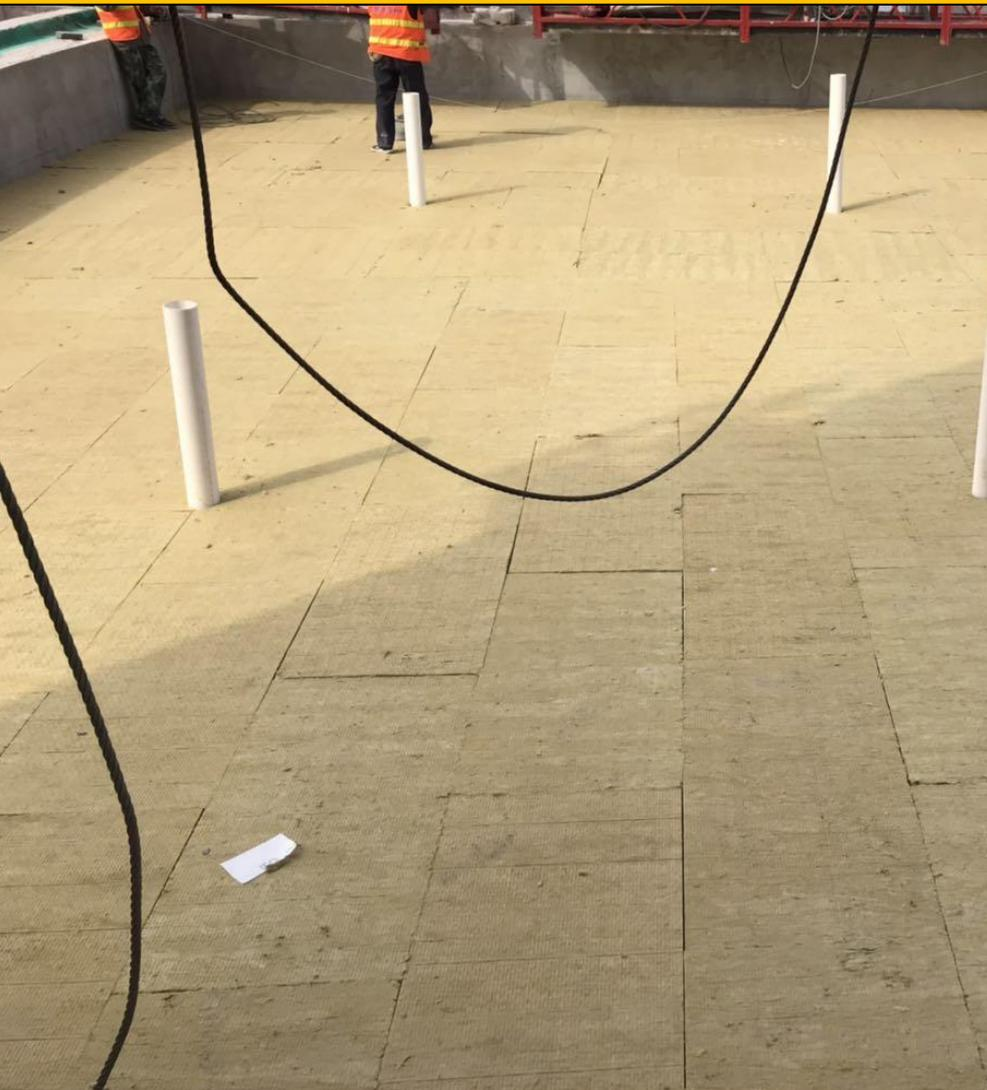
**Mockup room image** - Flat roofs at the top levels are insulated with XPS with a fire safety ring of mineral wool on the outer perimeter
