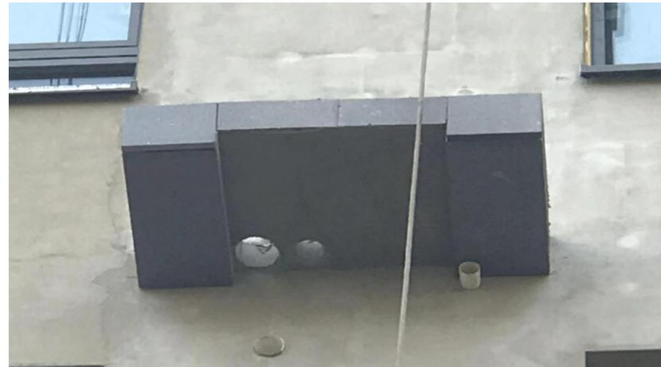
**Double beam technical balcony after installing the wall system**
