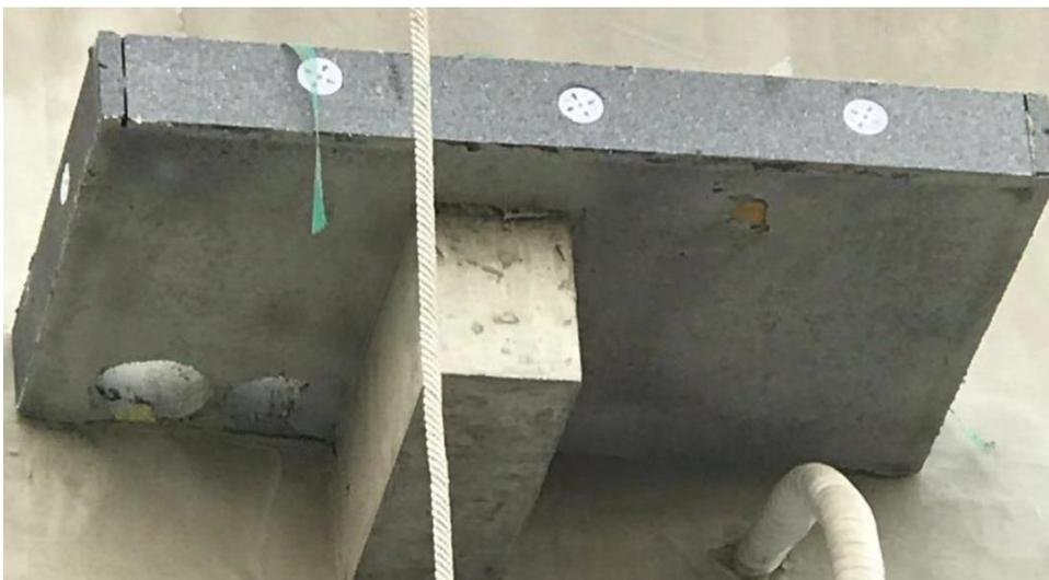
**Single beam technical balcony after installing the wall system**
