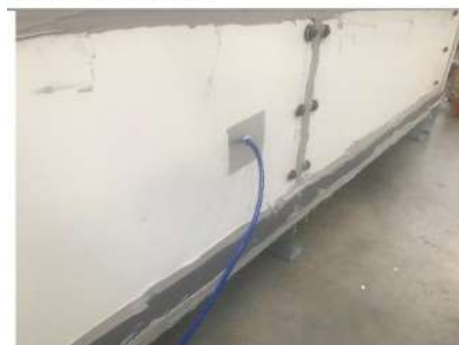
Inside pressure measuring point
