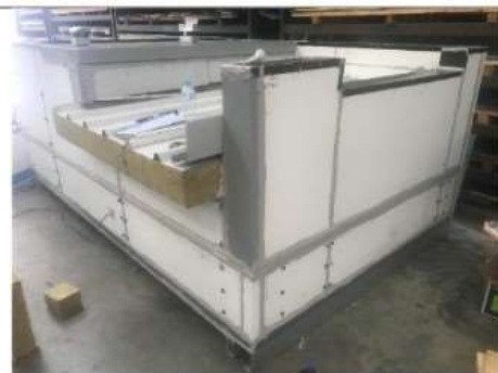
Roofing and box gutter sample of the mock-up
