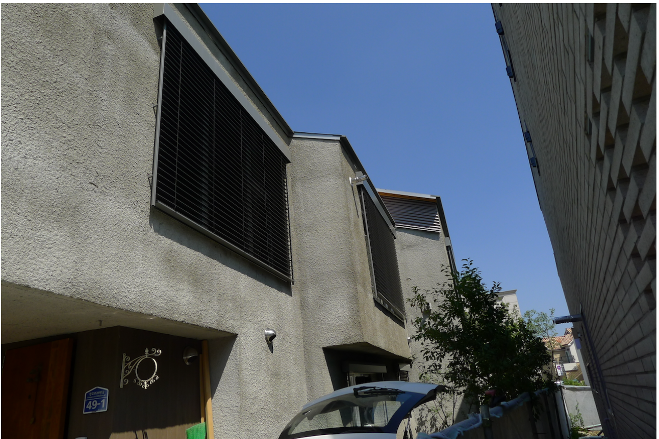
South-west side faces the neighbour house. It has big windows and external venetian blinds. There can be seen the outdoor air intake hood, the exhaust air outlet hood on the ground floor, and the flue terminal for the gas boiler on the first floor.
