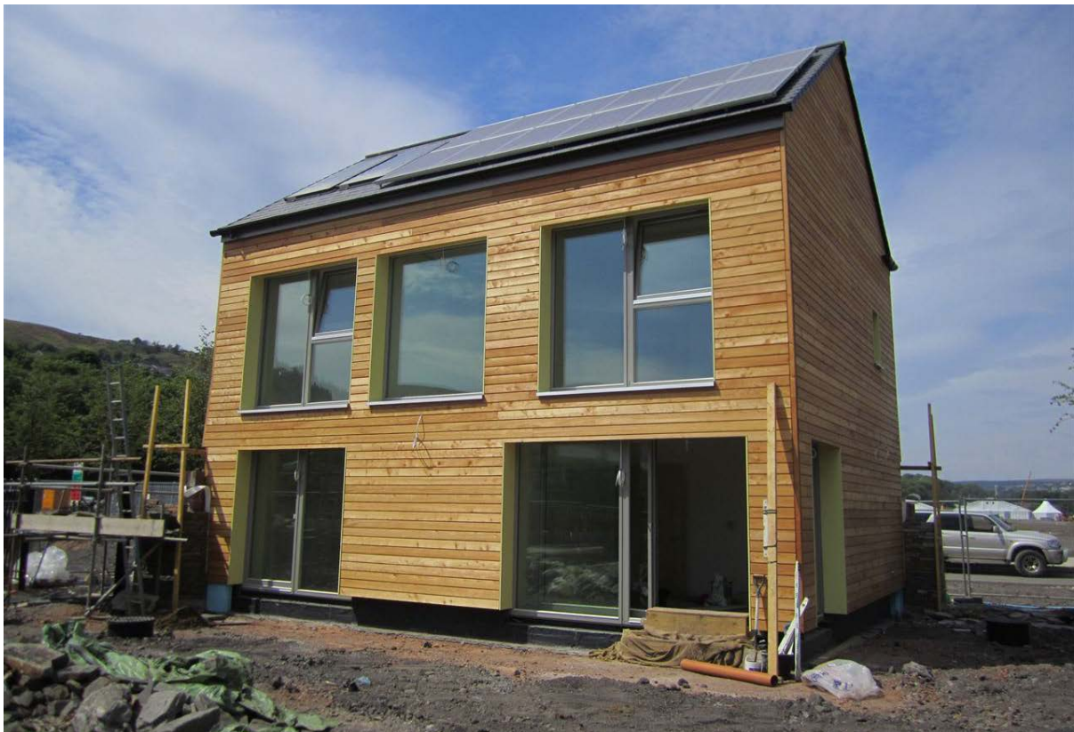
Figure 4. Image showing South and East Elevations of Larch House, under construction
