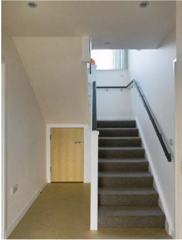
Figure 5. Image showing interior hallway, stairs and half landing
