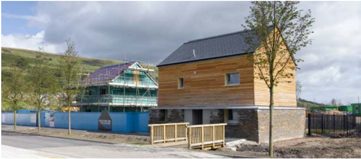
Figure 3. Image showing North and West elevations of Larch House
