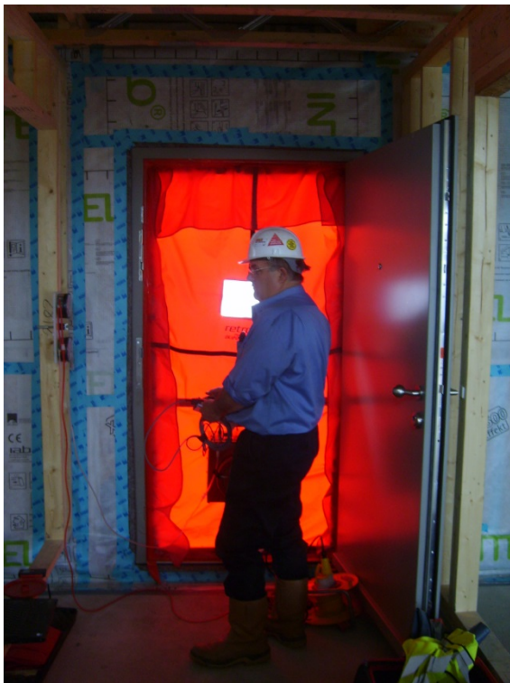
Figure 16. Interim blower door set-up for ATTMA (EN13829) pressure test
