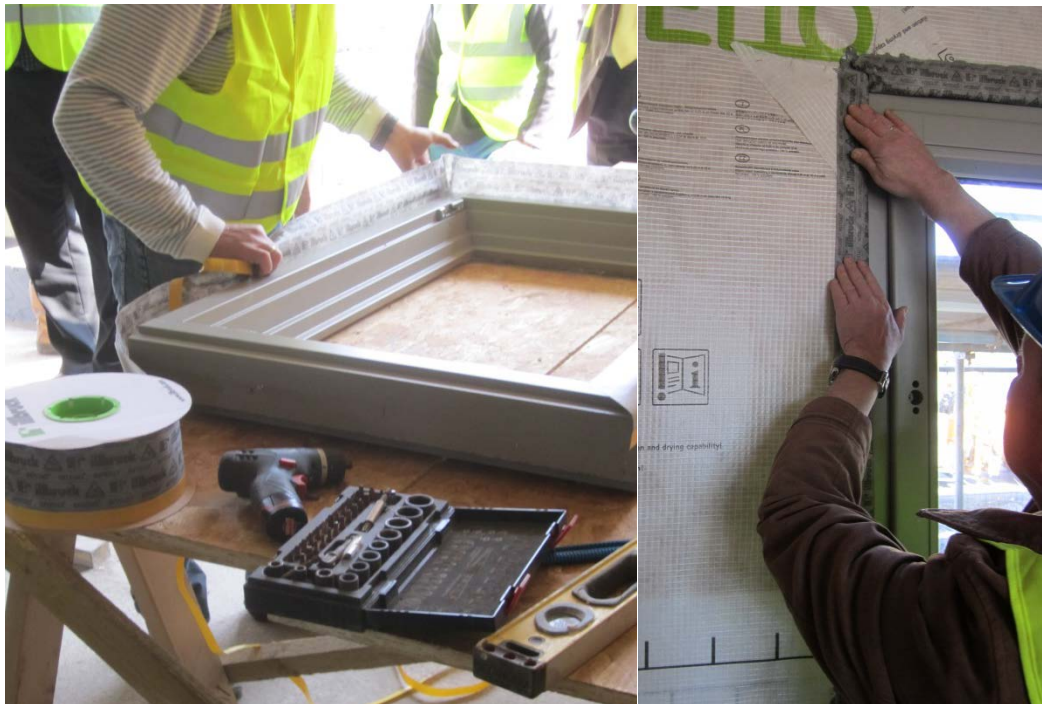
Figure 15. a) Pre-fitting of airtightness tapes b) installation taping connection to VBL
