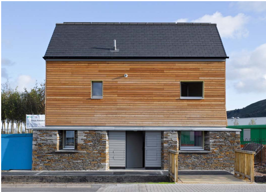
Figure 2. Image showing North elevation of Larch House
