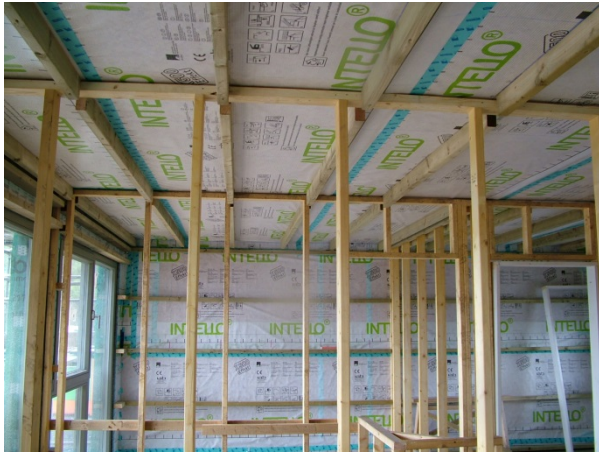
Figure 12. Internal wall and ceiling framing under construction
