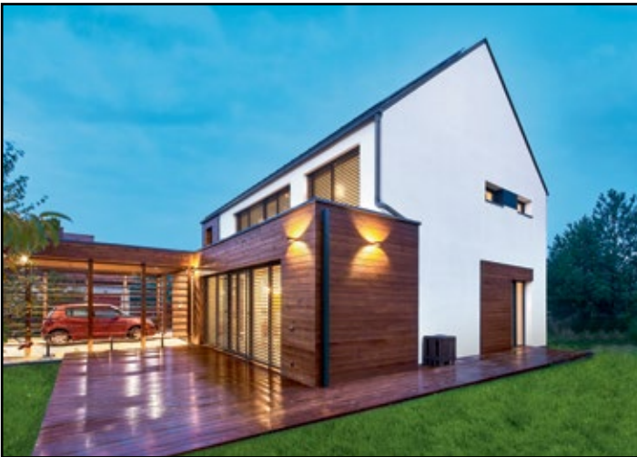
View of the south facade
