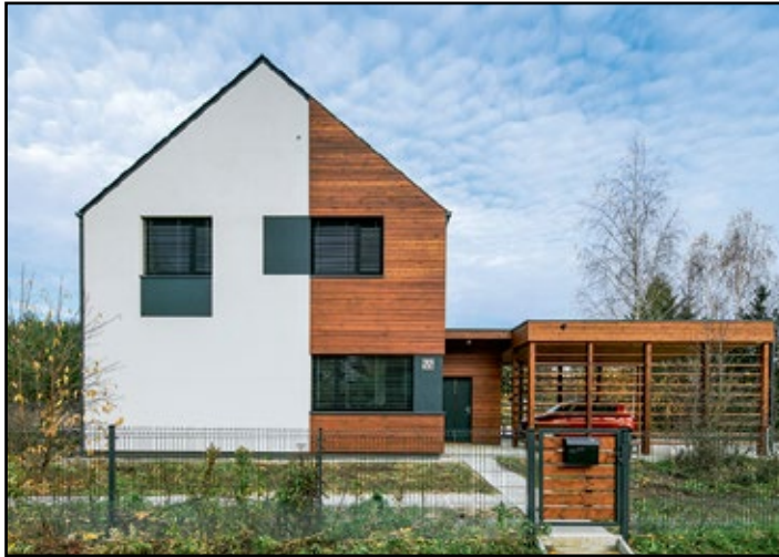
View of the west facade
