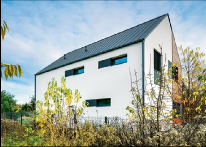
View of the north facade
