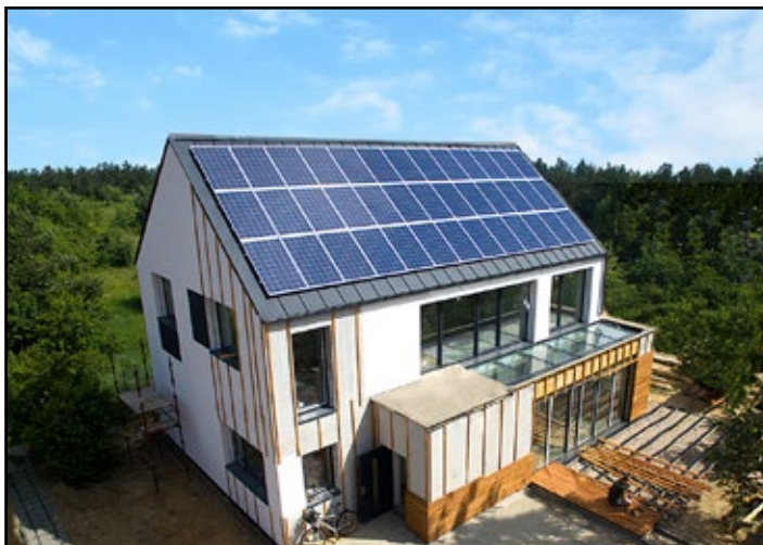
View of the building during construction period
