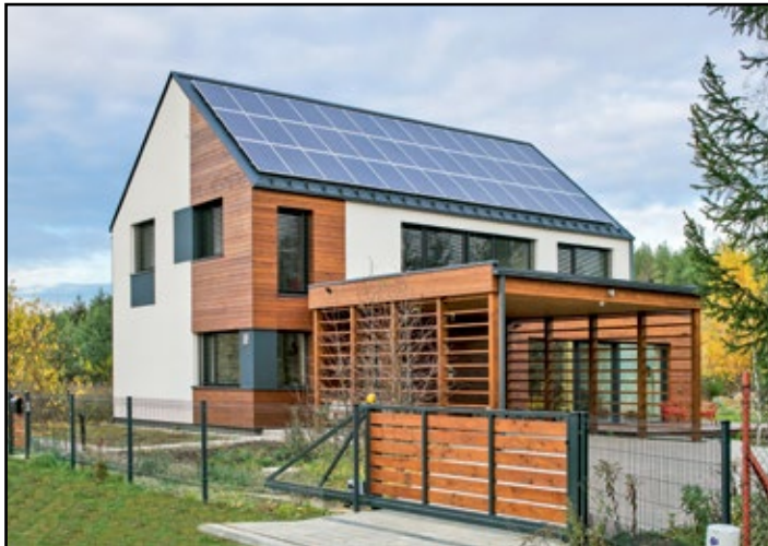
View of the south facade
