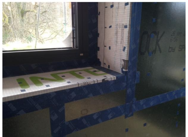
These 5 images show the thermal break in the structural timber frame with the insulation extending over the timber part of the window frame (top left); the Gutex installation at the exterior window frame (top right); the Gutex installation at the exterior window frame from side view (bottom left); the window sealed with flashing tape under the aluminium sill (middle right); the internal airtight membrane and taping of the window installation prior to insulation in the reveal (bottom right).
