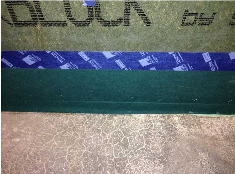
Where internal stud walls intersected with the external wall, or where the intermediate floor sat on top of the ground floor wall head, we installed strips of Pro Clima Intello Plus airtight membrane during the timber frame assembly to ensure we could get continuity of the airtight barrier once the external frame was wind and water-tight.
