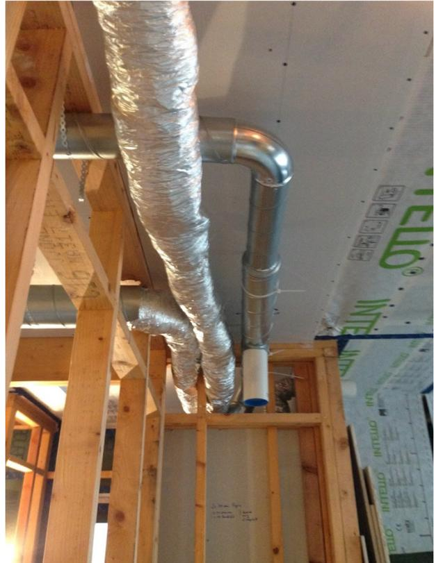
These photos show the ducts being installed. The insulated semi-rigid ducts sleeved over the hallways (top left); a silencer on the rigid duct system (bottom left); the combination of rigid and semi-rigid ducts (right).
