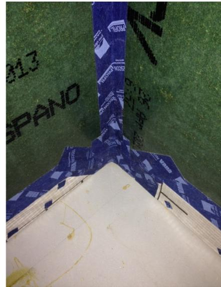
These 4 images show the thermal break in the timber frame wall construction (top left); the internal vapour control and airtightness board, which also served a structural purpose (top right); the airtight seal between ground floor wall and concrete slab (bottom left); the airtight seal around the intermediate floor at the bottom of the first floor wall panel (bottom right).
