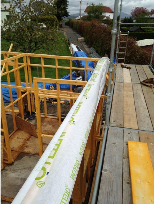
Once the first floor chipboard deck was installed the membrane was pulled back towards the inside of the frame and taped to the Vapourblock board on the first floor walls.
