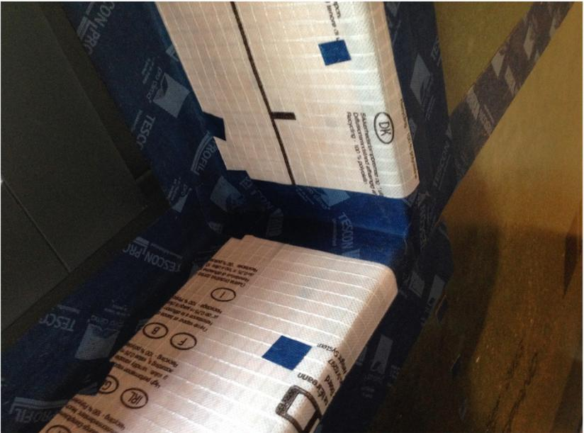
The first floor ceiling was covered in a layer of the same Intello Plus membrane, and taped to the top of the Vapourblock board on the first floor walls.
