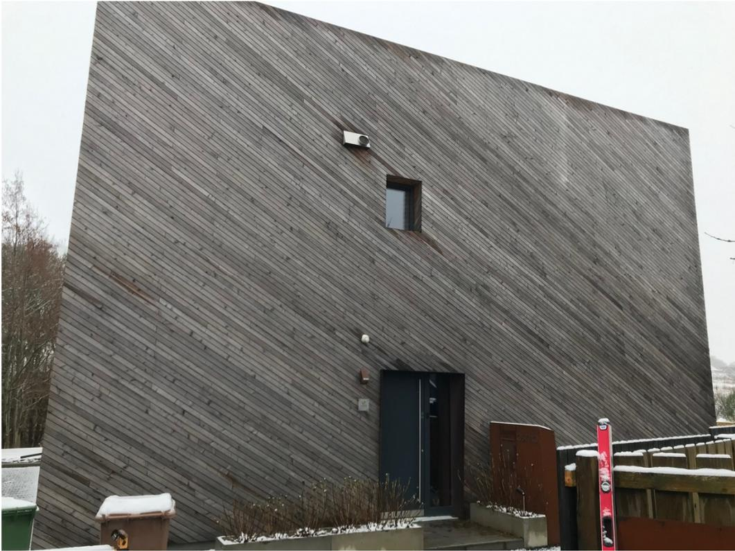
The North Elevation of Ostro Passivhaus. The MVHR grille can be seen at first floor level. This elevation has minimal openings.
