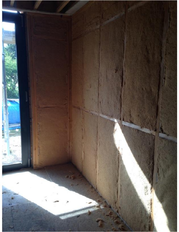
These 4 images show the insulation of the timber frame. The double height 245mm studs being insulated (top left); the parapet inner frame being insulated (bottom left); the overinsulation at the window frames (top right); and the fully filled insulated ground floor wall (bottom right).
