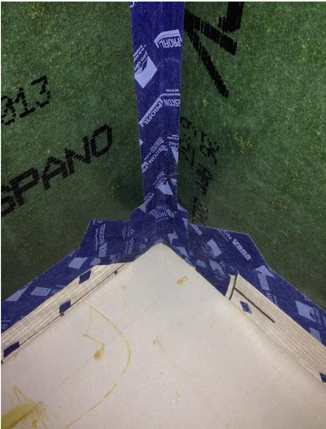
This airtight layer was then extended into the window, door and rooflight reveals using Pro Clima Intello Plus membrane, and again all connections, joints and staples taped using Tescon Vana tape.
