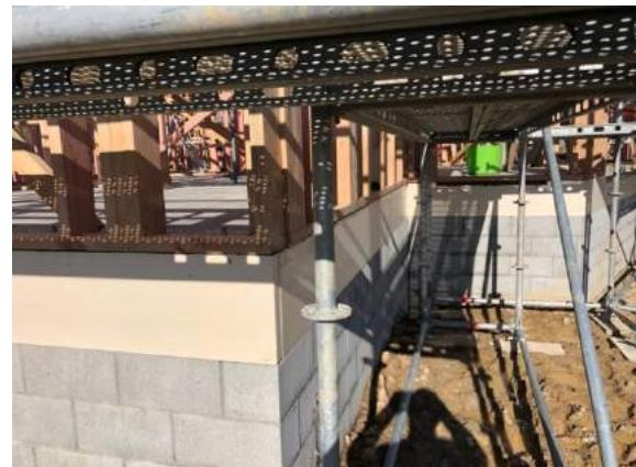
Framing cantilevered over edge insulation
