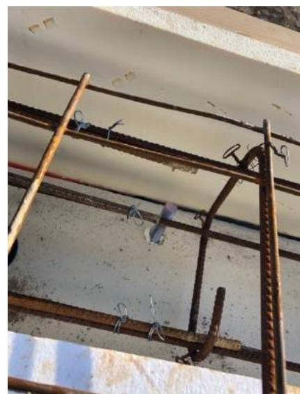
Slab edge thickening construction
