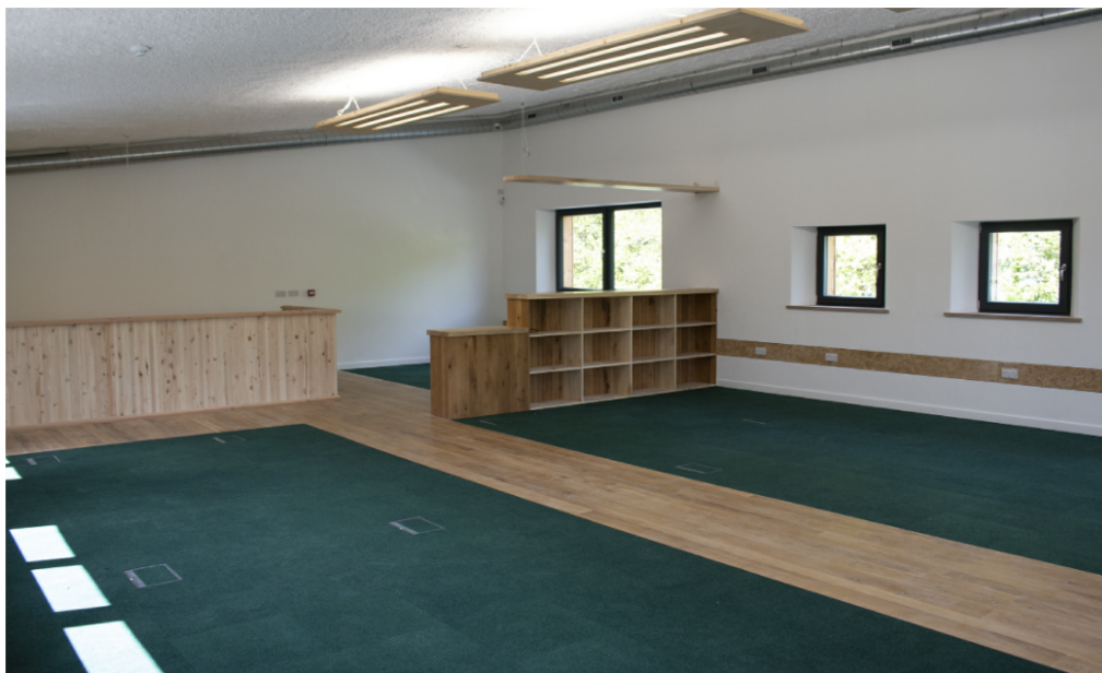
Figure 32 – Steel spiral wound ducting to first floor office
