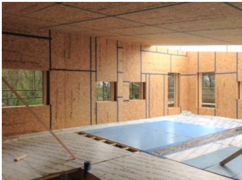
Figure 19 – Roof panels being erected
