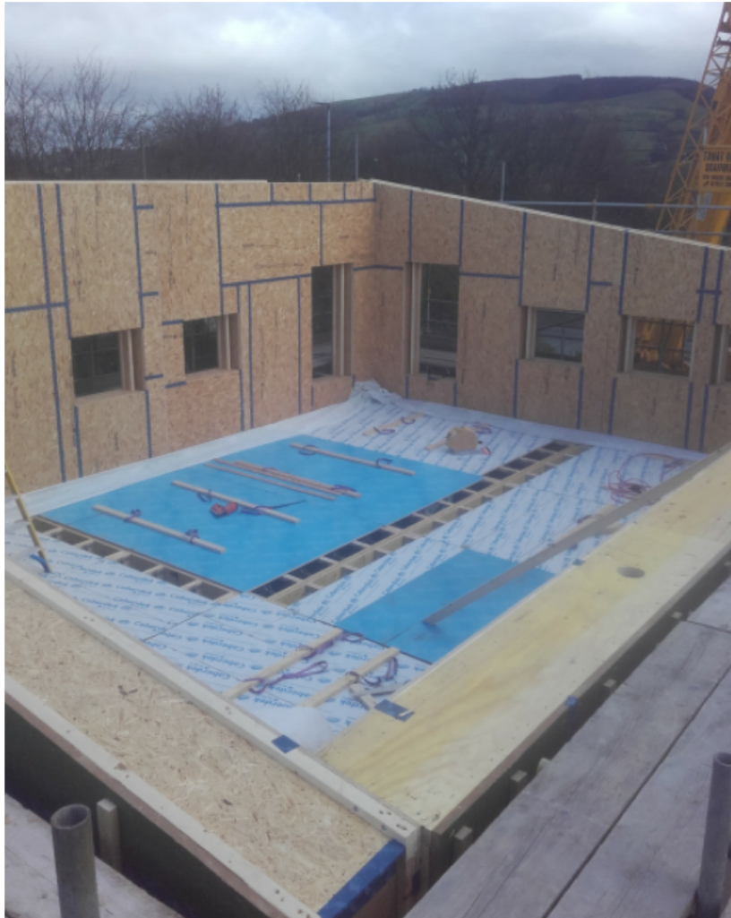
Figure 18 – First floor panels erected, showing eaves detail
