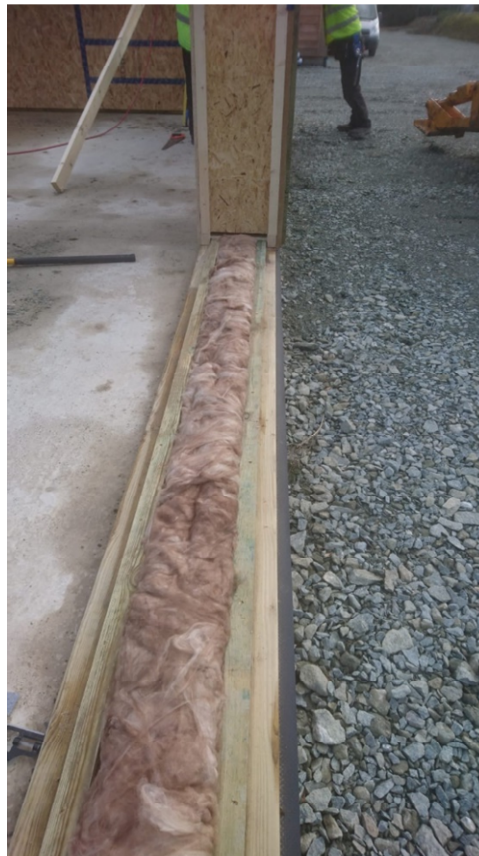
Figure 11 - Shows soleplate installation detail to the concrete slab
