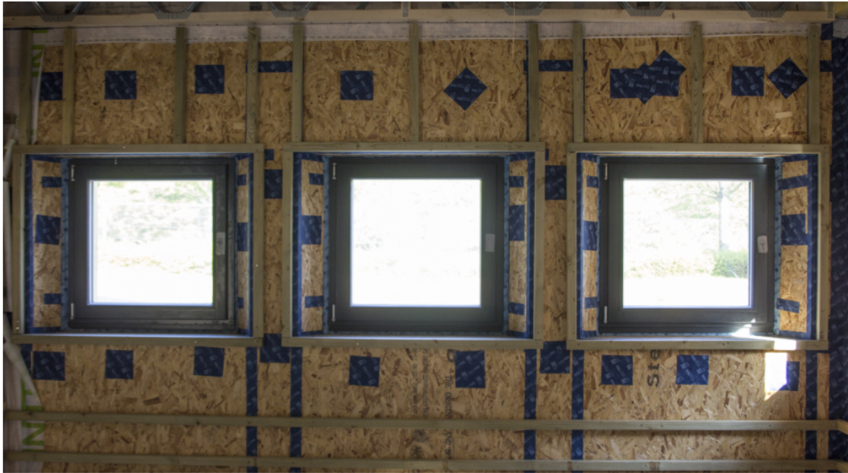
Figure 25 – Airtightness layer via OSB board and airtight tape
