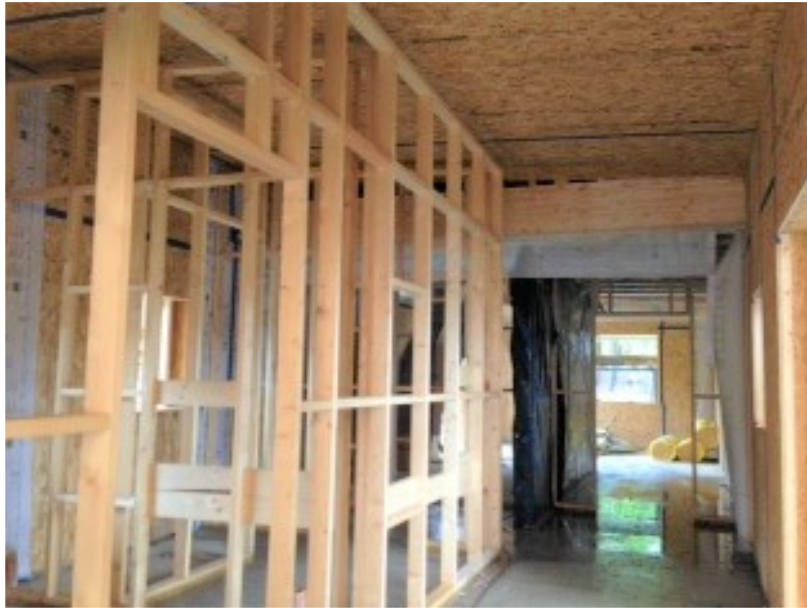
Figure 21 – Glulam beams supporting first floor roof (abutment)
