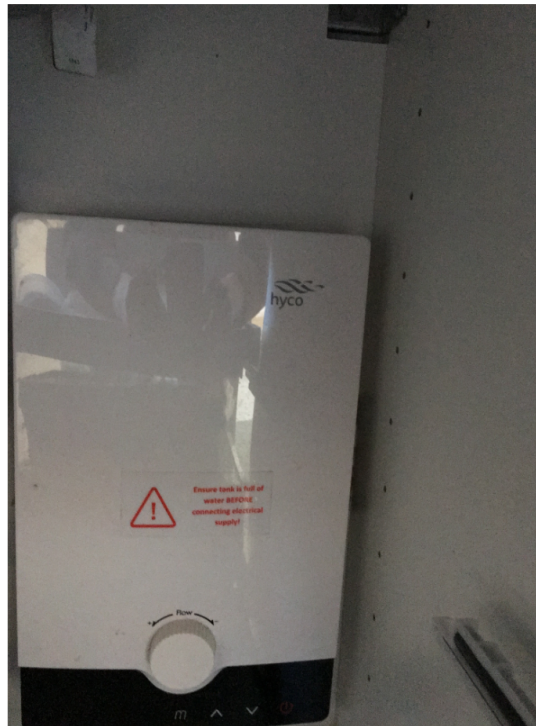
Figure 34 – Instantaneous water heater in location
