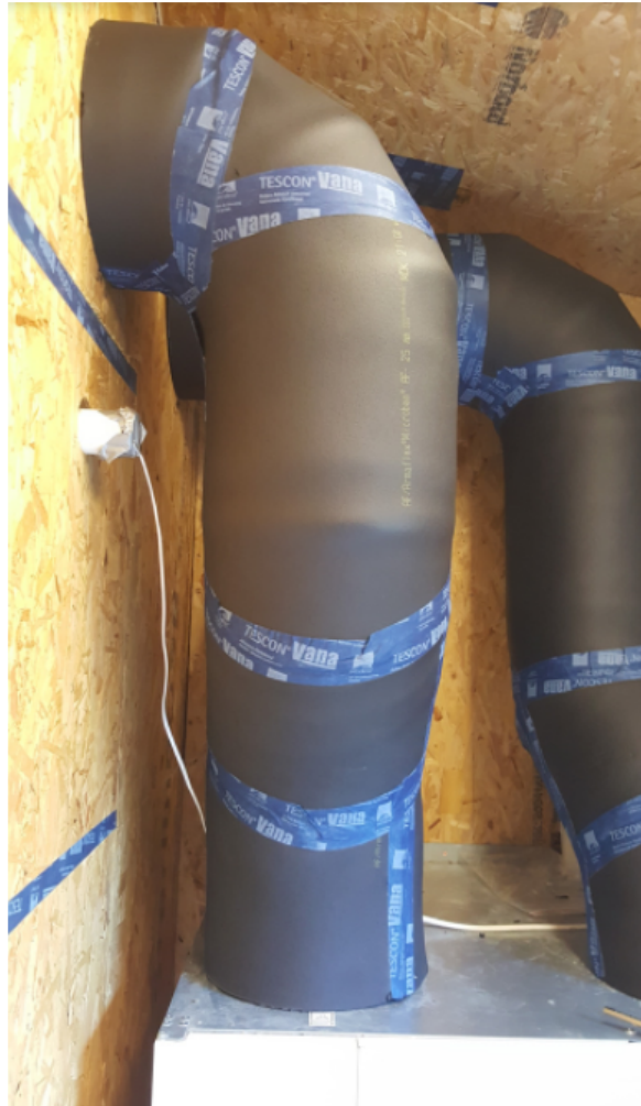
Figure 31 – Insulation to MVHR exhaust ducts
