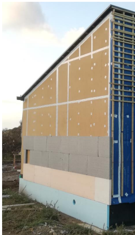
Exterior insulation starts in the footing
