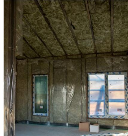
Timber framing with insulation between wooden studs
