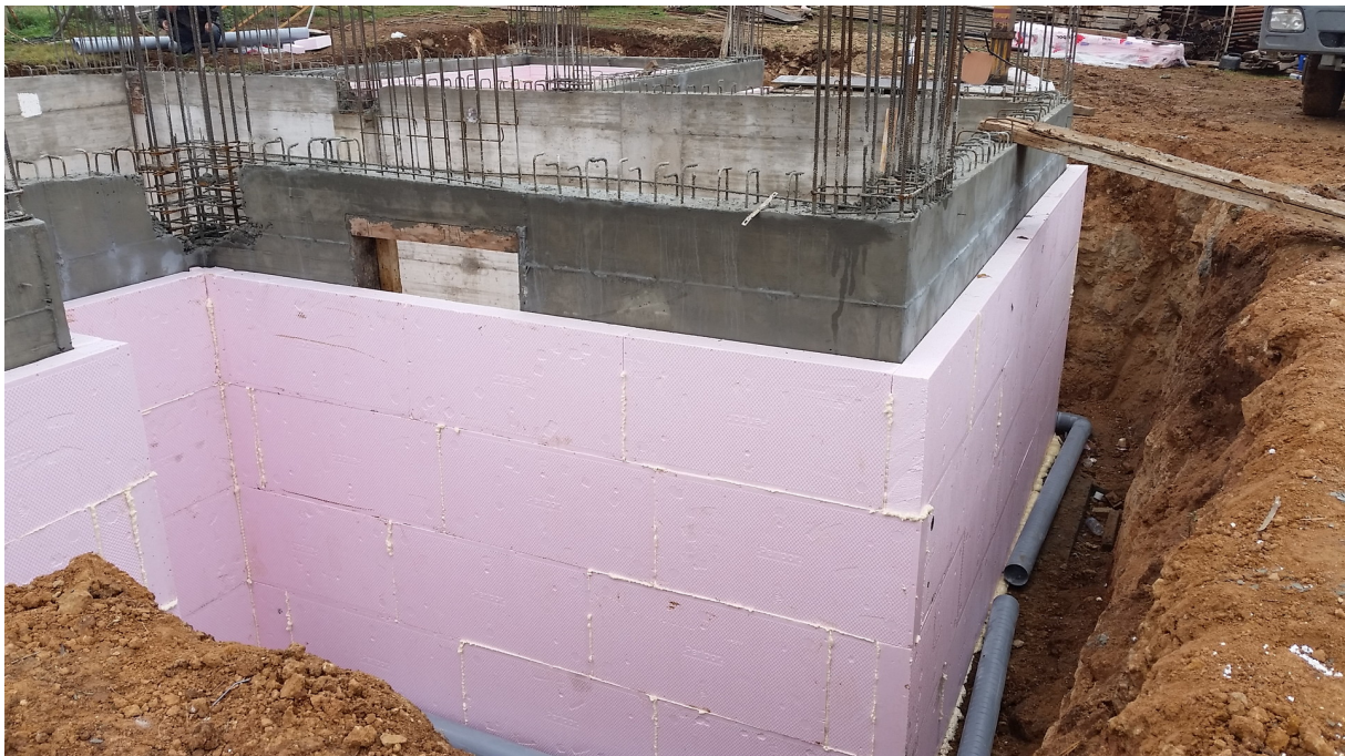
Picture 99. Basement wall insulation
