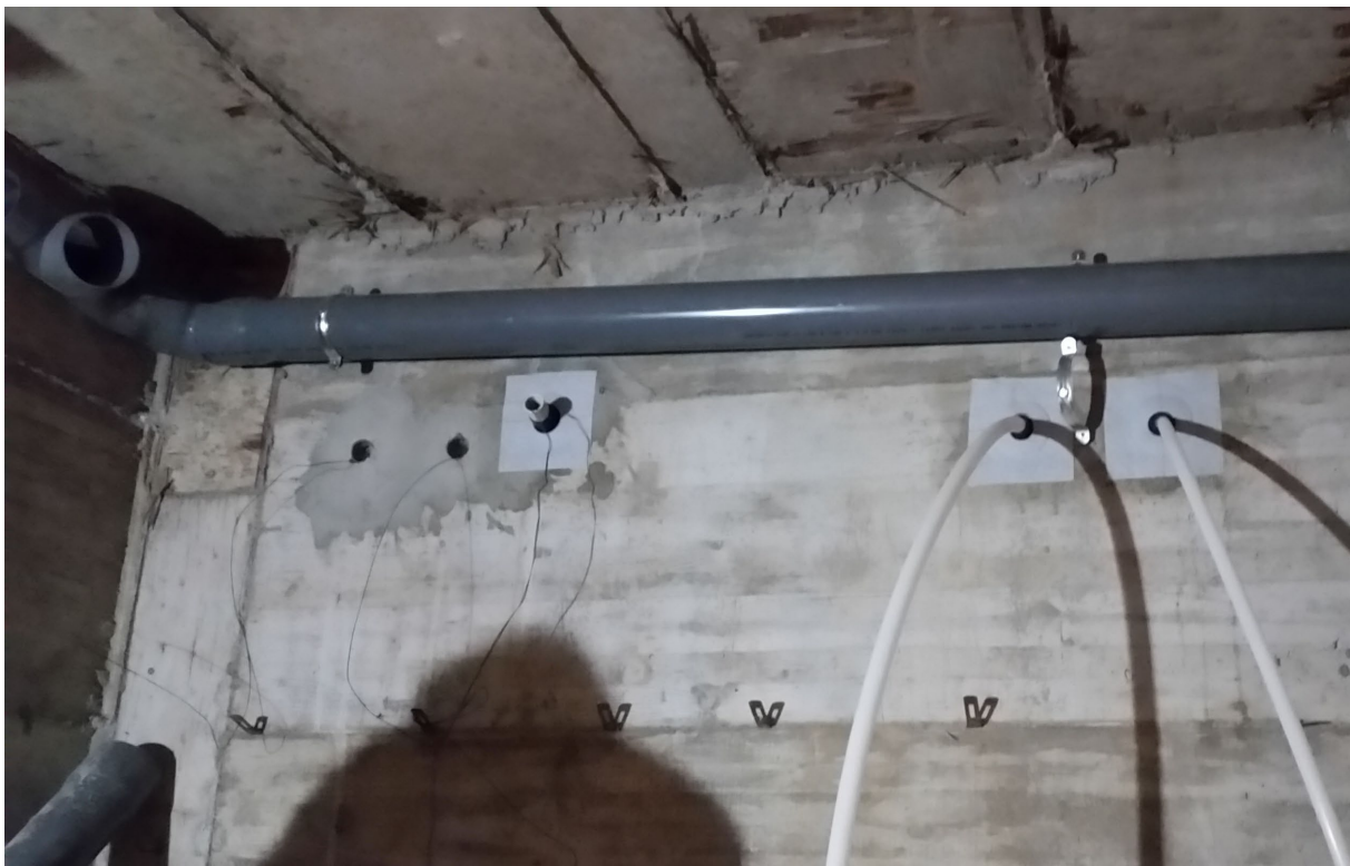
Picture 20. Sealing collars on ducts
