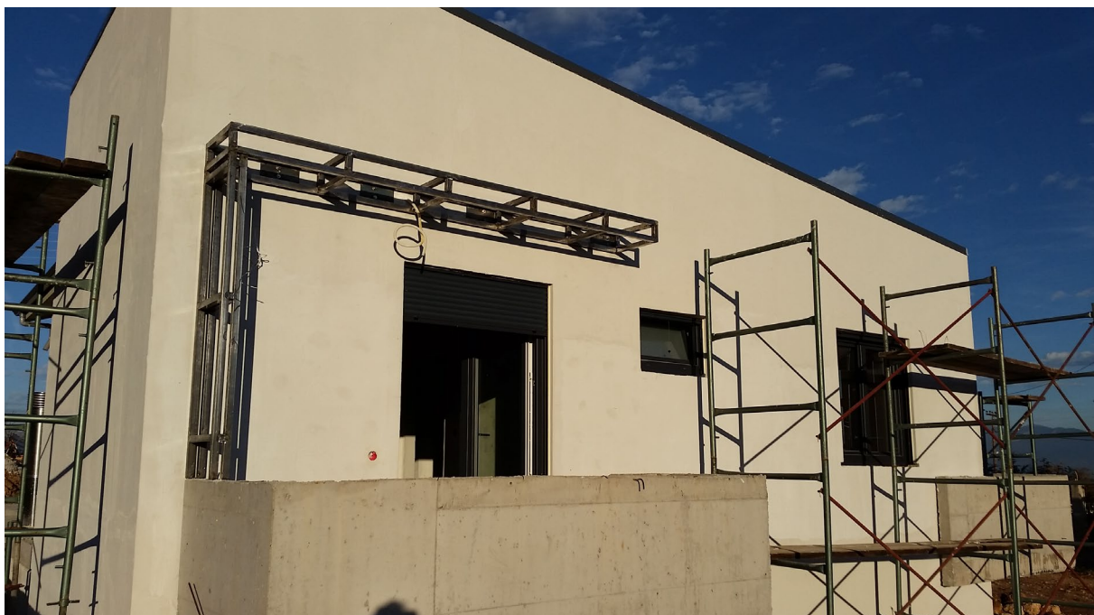
Picture 15. Shading construction
