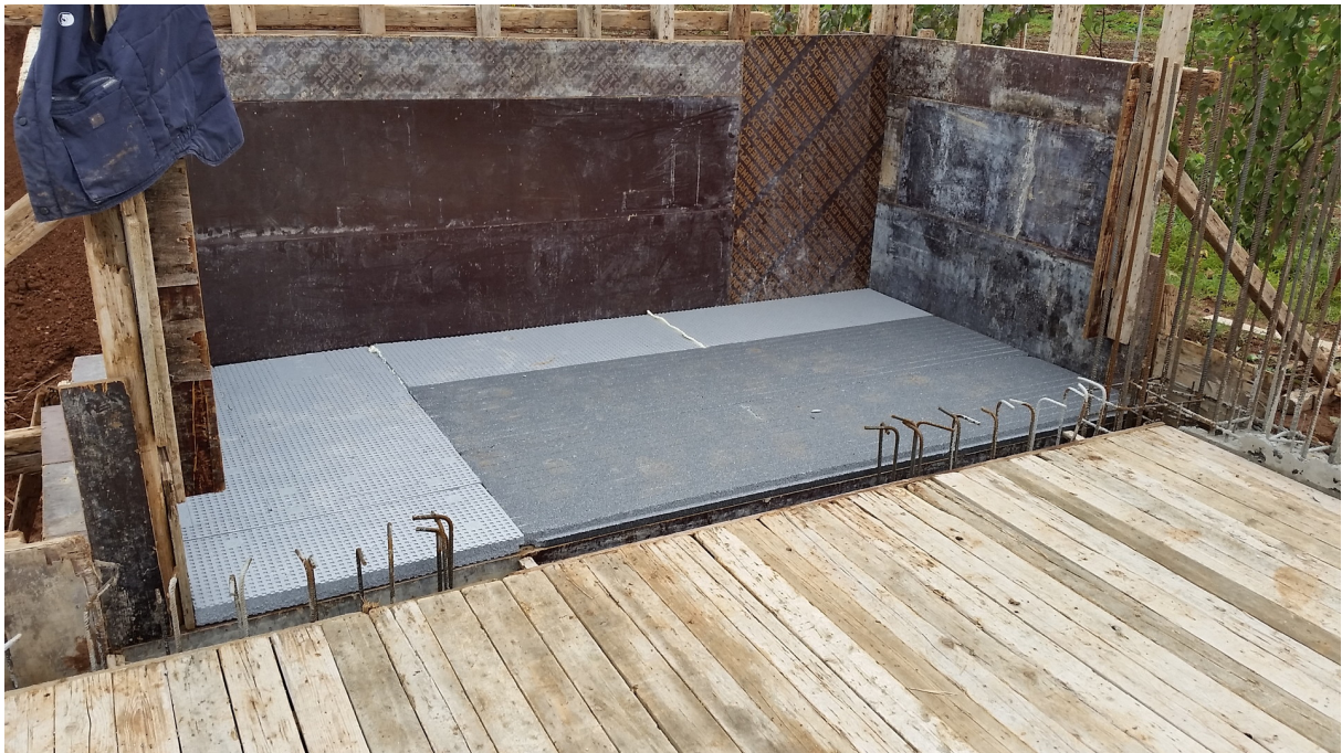
Picture 13. Balcony insulation
