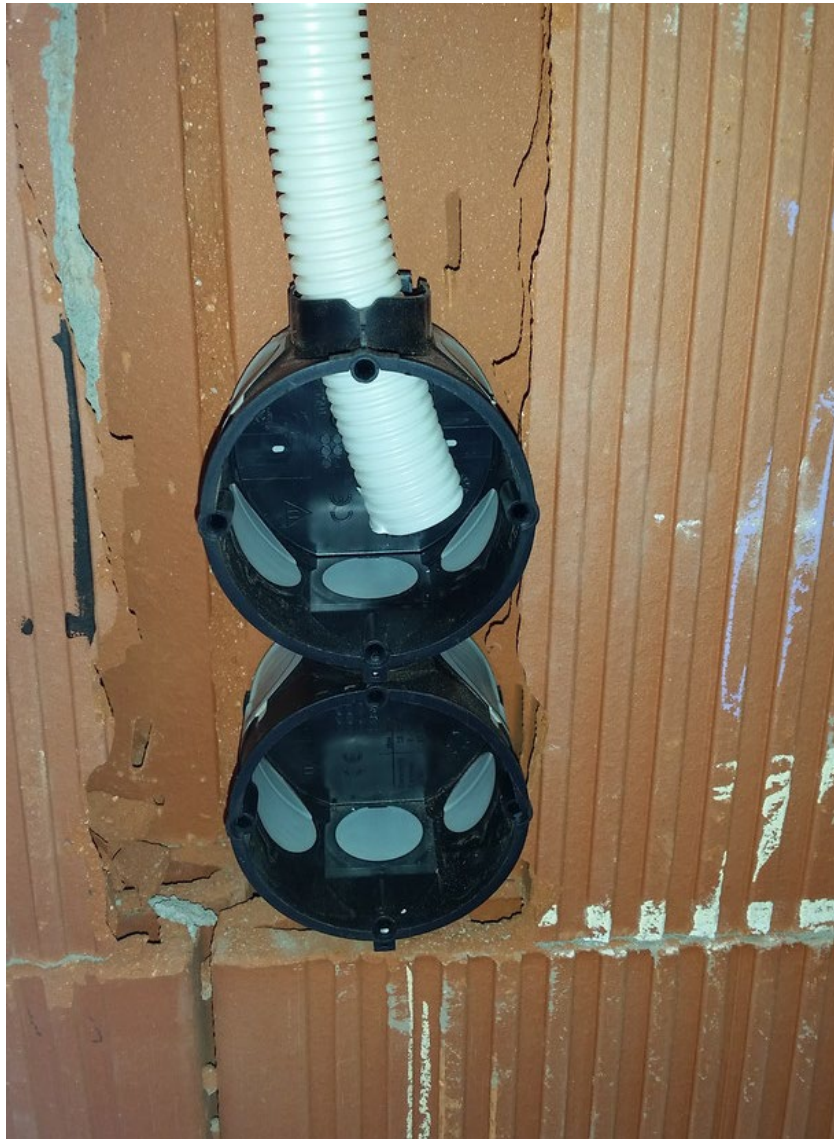
Picture 21. Airtight electrical junction boxes
