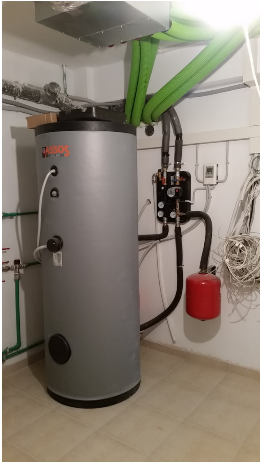
Picture 28. DHW installation
