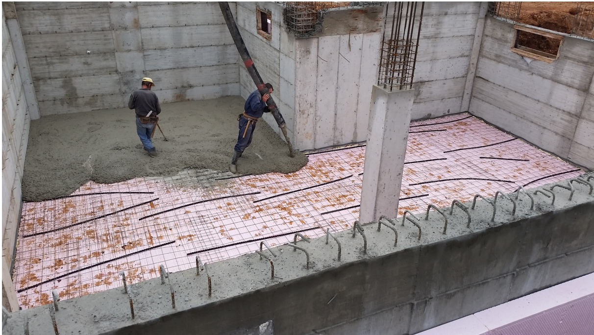
Picture 10. Placement of insulation below the basement floor slab
