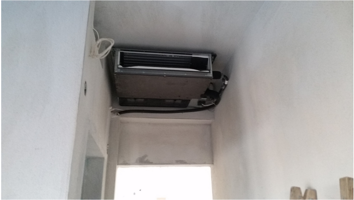
Picture 26. Split unit air condition
