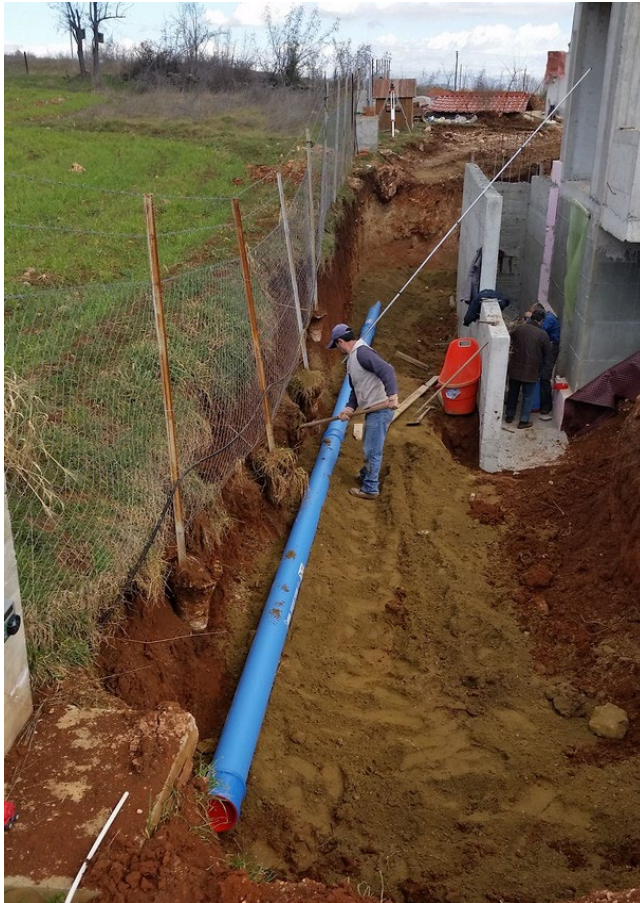
Picture 24. Geothermal heat exchanger
