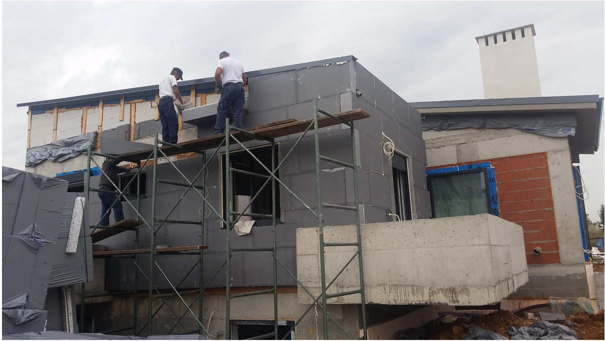
Picture 8. Placement of the exterior insulation of the thermal envelope
