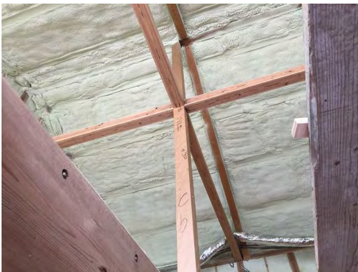
Thermal insulation work for wall Urethanform: t=150\text{mm}
