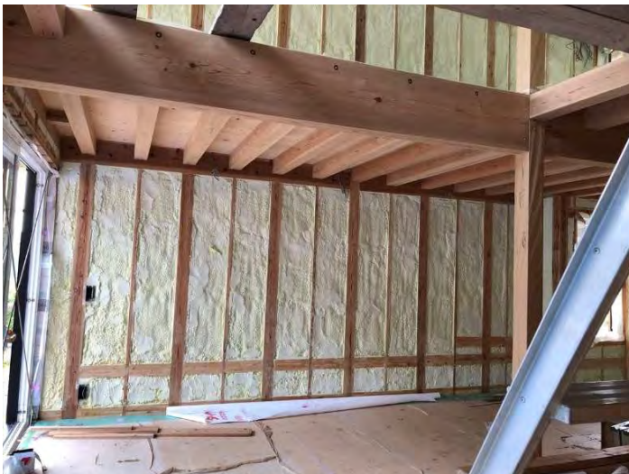
Thermal insulation work for wall Urethanform: t=90\text{mm}
