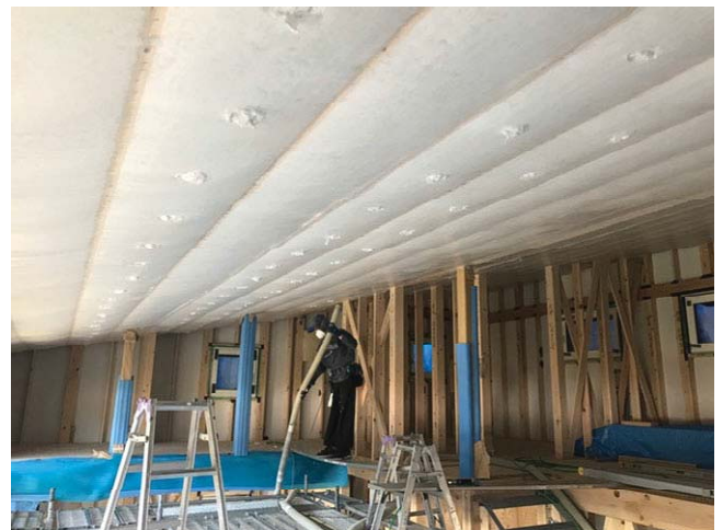
充填 Blowing glass wool 施工状況
