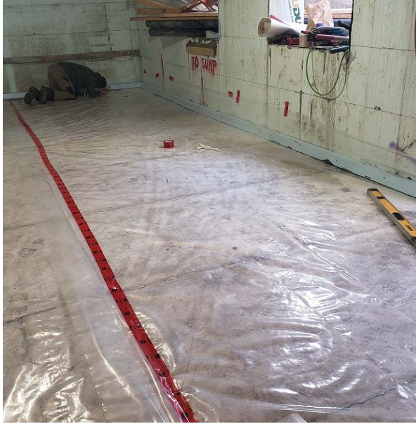
Poly sheet air-vapour barrier under concrete slab with additional EPS thermal break at slab edge
