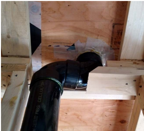
Typical plumbing vent penetration tape sealed
