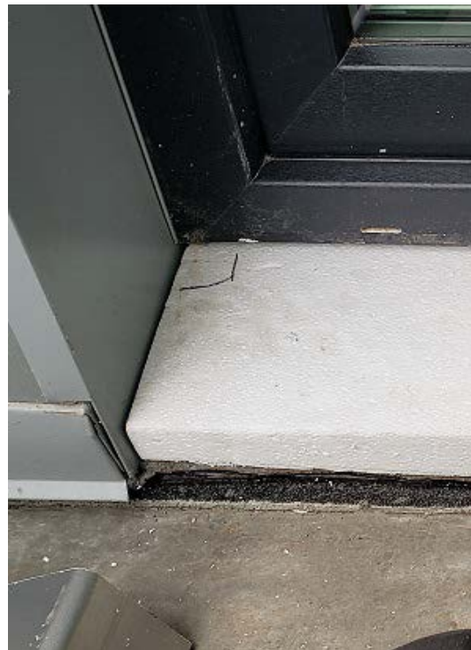
Tapered insulation at exterior door sill below stainless steel threshold
