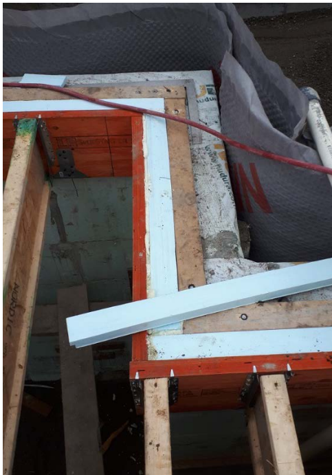
Main floor-ICF wall junction Note EPS insulation filler behind LVL ledger
