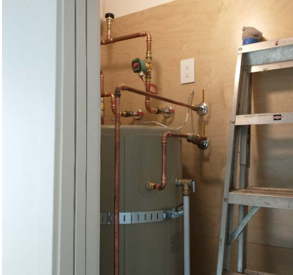
Sanden model SAN-83SSAQA DHW Tank
