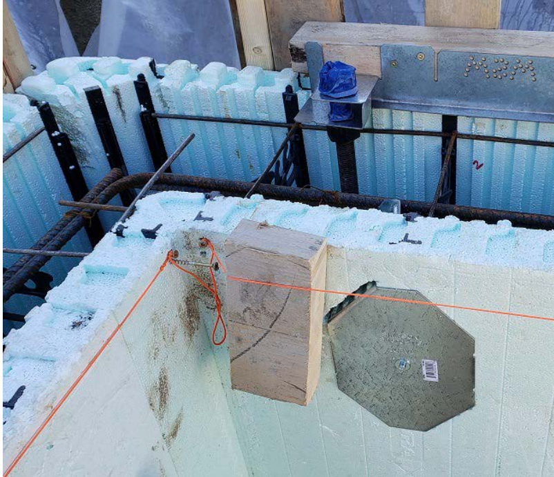
ICF wall corner detail
