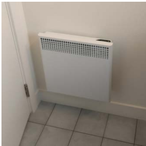
Typical electric wall heater
