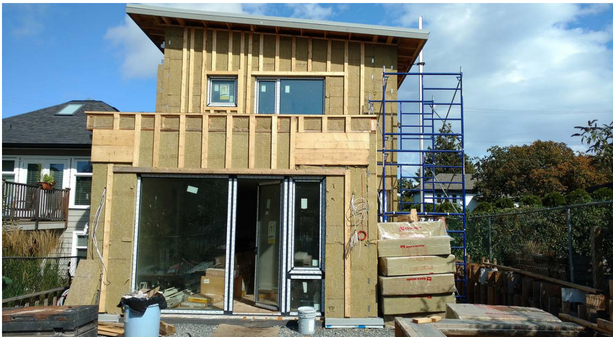
Exterior insulation & strapping secured to ACS ties. Note wood blocking for awning attachment placed within strapping layer to eliminate thermal bridging.
