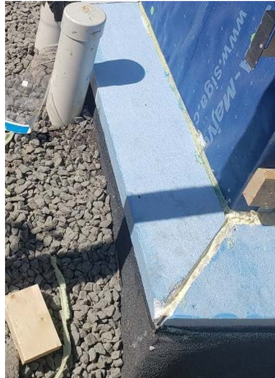
ICF-frame wall junction with tapered XPS
