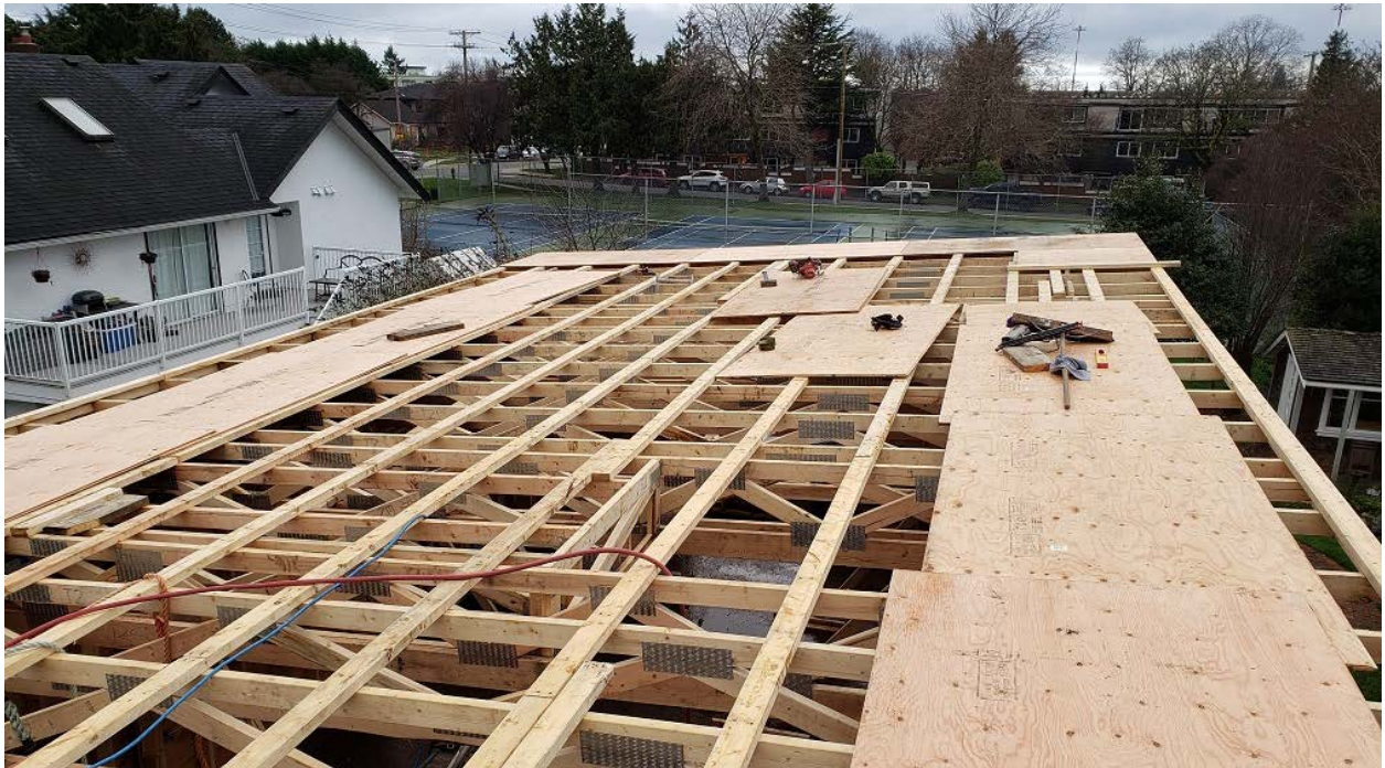
Upper level sloped roof trusses. Note 38x89 cross strapping for roof ventilation.
