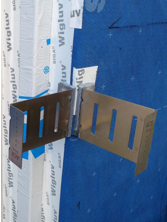
ACS stainless steel wall ties w/ Proloft aerogel thermal break
