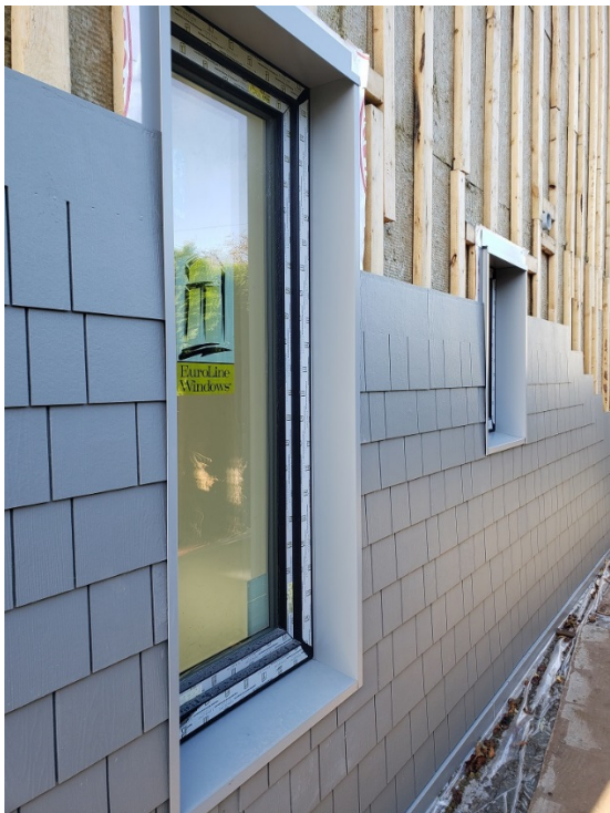
Typical metal window sill & trim at frame wall
