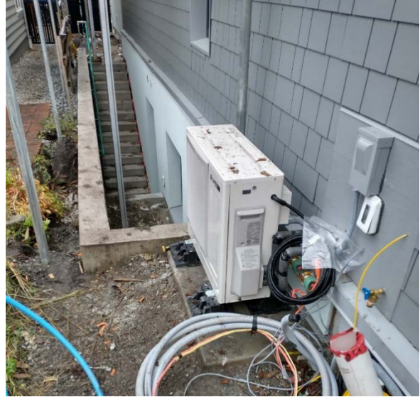
Sanden DHW Heat Pump model GUS-A45HPA
