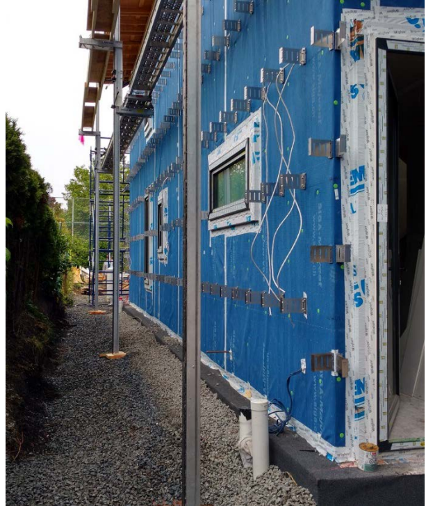
Tie spacing 406mm oc hor & 812mm oc vertical Note SBS waterproofing over top of ICF wall
