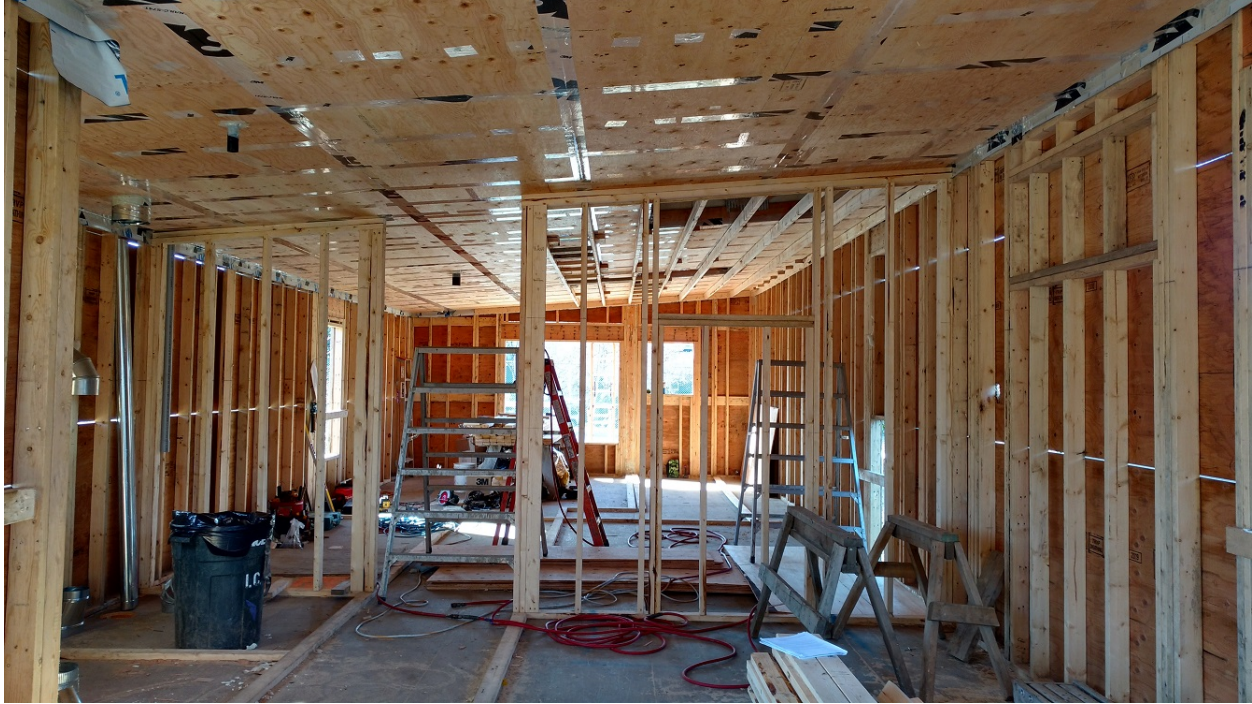
Upper level roof plywood air barrier with taped joints at underside of wood trusses. Note self-adhered membrane flashing transition to exterior Siga Majvest over top wall plate. Note 2x4 ceiling framing being installed at rear for insulated cavity to house electrical services & HRV ducts below plywood.
