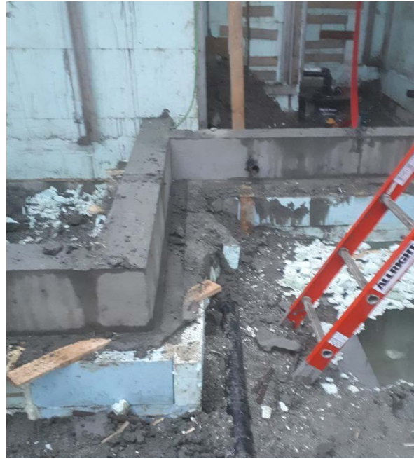
Interior shear wall foundation. Note rigid insulation below and each side of concrete footing.
