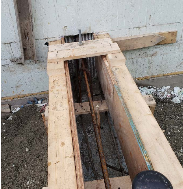
Interior shear wall foundation. Note rigid insulation below and each side of concrete footing.
