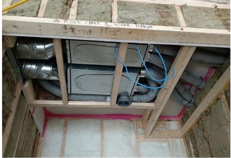
Zehnder manifold-silencers, sheet metal & ComfoFlex ducts
