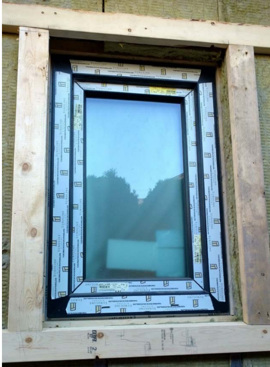
Window & strapping surround in frame wall
