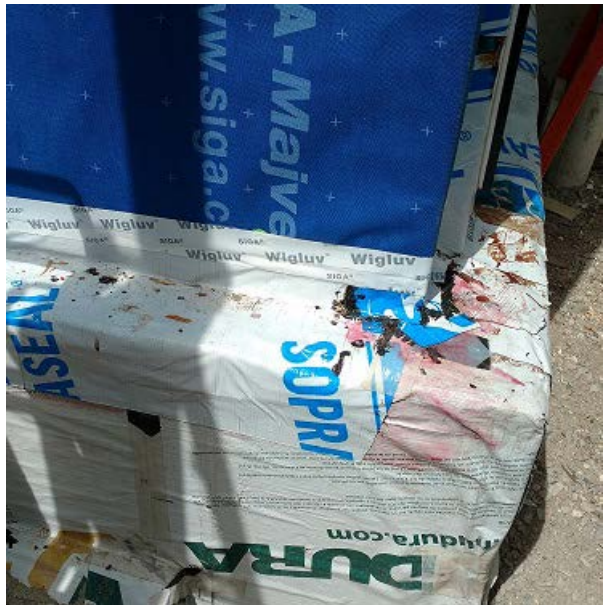
Self-adhered membrane (SAM) air barrier at ICF to wood frame wall transition
