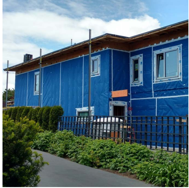
Siga Majvest air barrier with Wigluv taped joints
