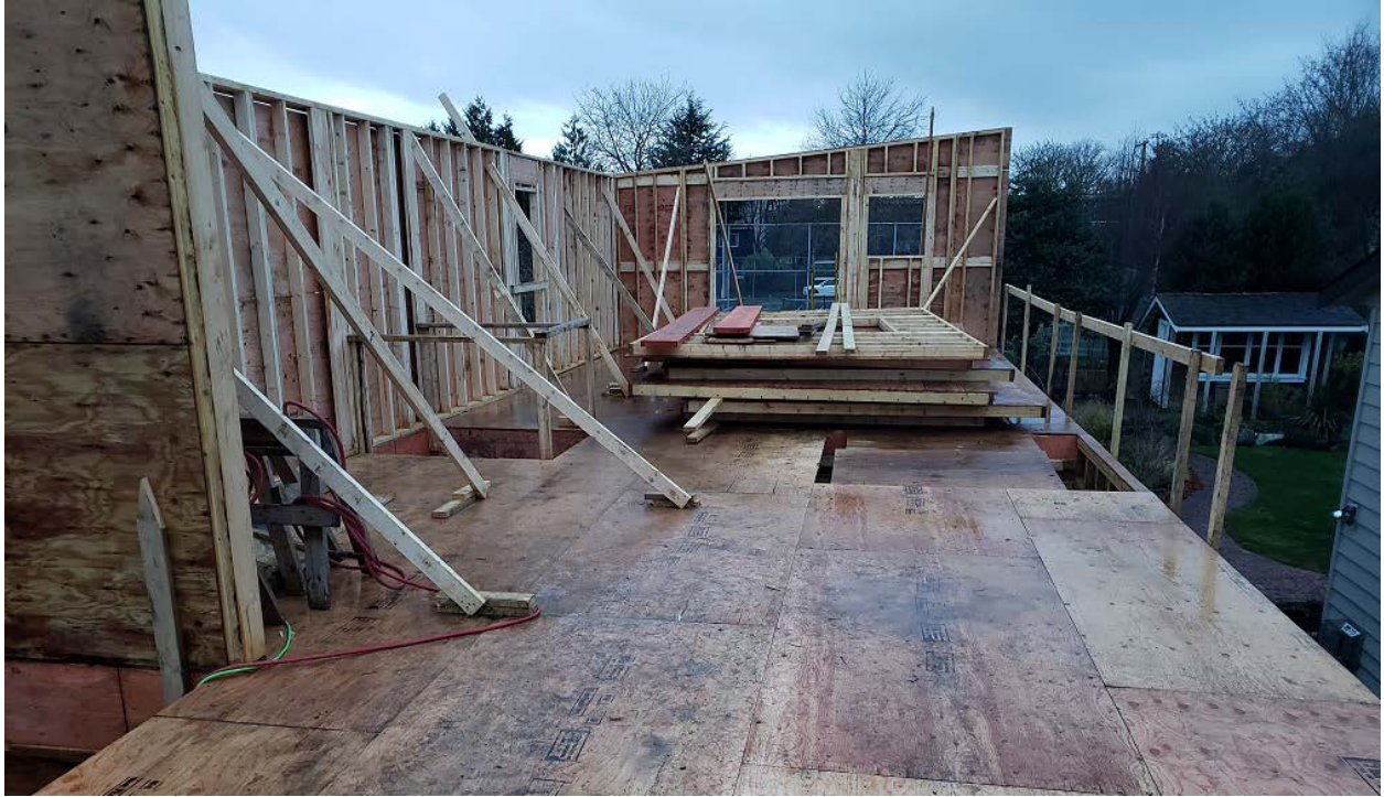
Typical prefabricated exterior wall wood frame panels
