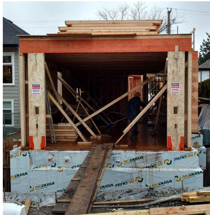
South wall shear frame in wall at LR opening
