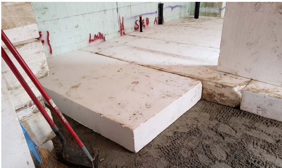
EPS Insulation on sand bedding & compacted fill under basement floor slab
