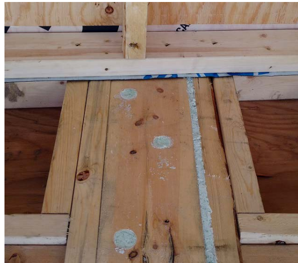
Exterior wall to service cavity framing. Note spray foam insulation used to fill framing gaps & voids.
