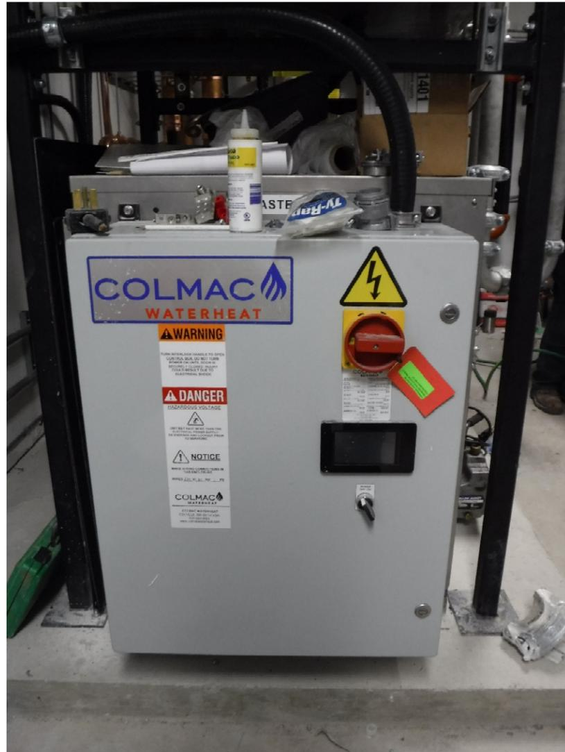
*COLMAC WATER SOURCE HEAT PUMPS WERE USED TO PROVIDE SERVICE WATER HEATING.*
