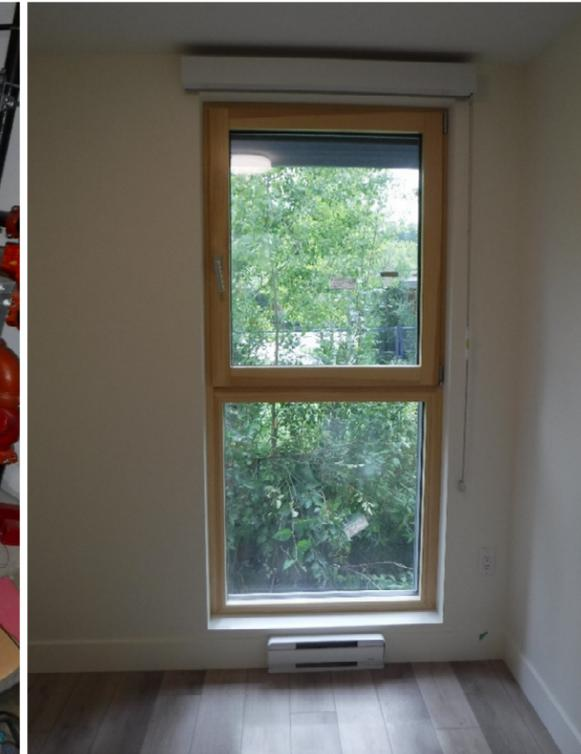
WATER SOURCE VRF HEAT PUMP PROVIDES SPACE CONDITIONING THROUGH THE YEAR. (LEFT) IN SUITE ELECTRIC BASEBOARDS ARE PROVIDED FOR TOP UP HEATING. (RIGHT)
