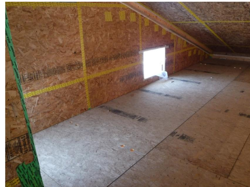
TAPED OSB FORMS THE MAIN AIR BARRIER ON THE WALLS AND ROOF ASSEMBLY.
