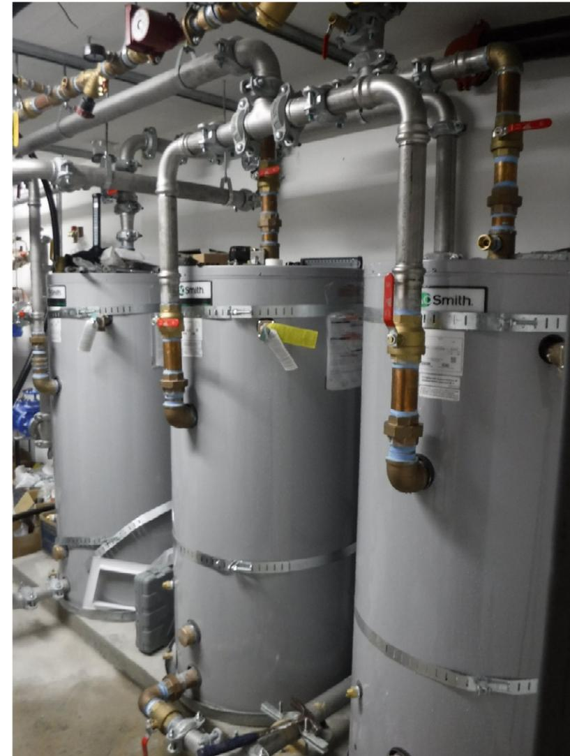
*THREE SERVICE WATER HEATING STORAGE TANKS WITH THERMAL JACKETS.*
