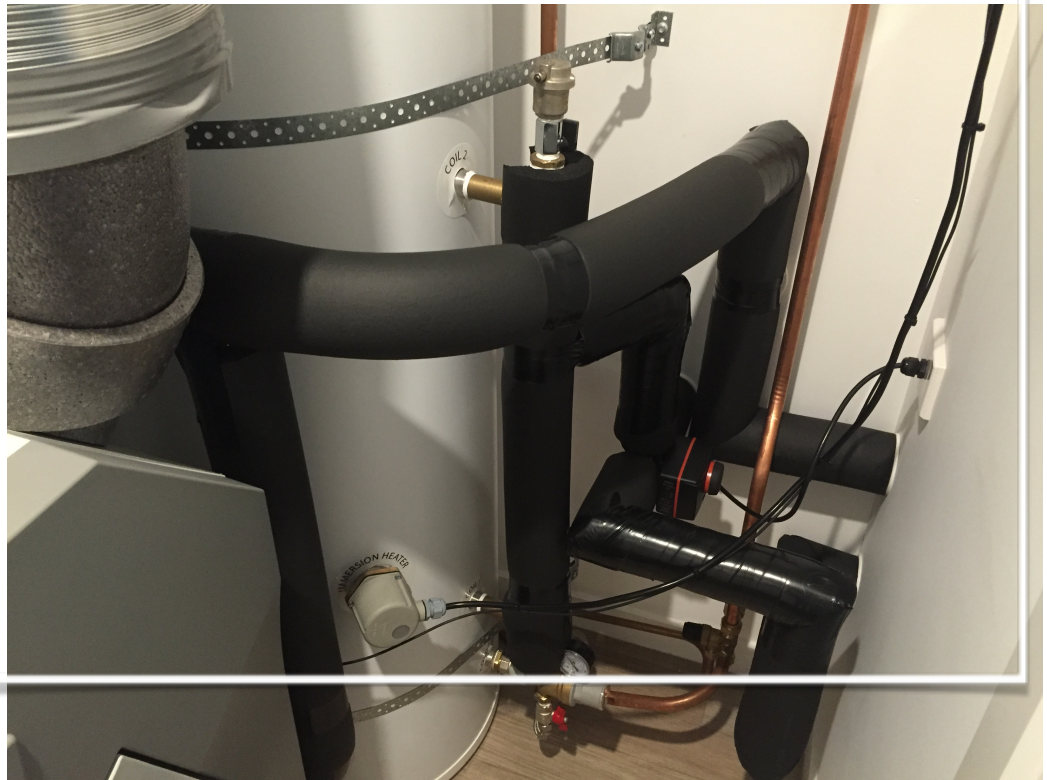
The Zehnder CombiAir 350 and hot water cylinder in the service cupboard
