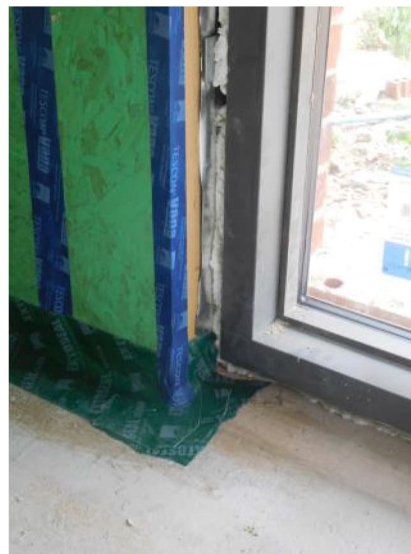
Figure 20: Airtightness connection between wall and floor
