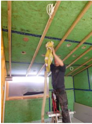
Figure 21: Warmcell insulation blown into roof cavity
