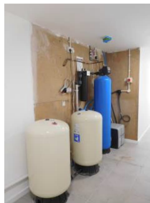
Figure 26: Borehole water purification unit
