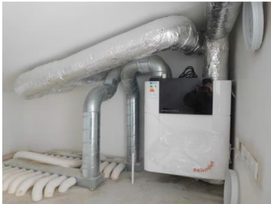
Figure 31: Zehnder MVHR unit
