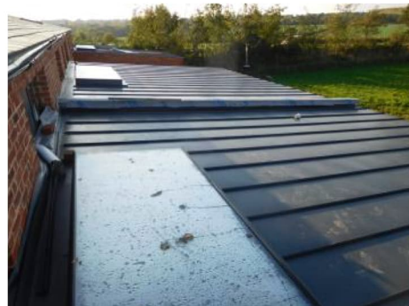
Figure 24: Standing seam metal covering to rear roof with 3m long rooflight
