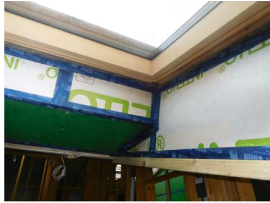
Figure 22: Airtightness detailing around rooflight
