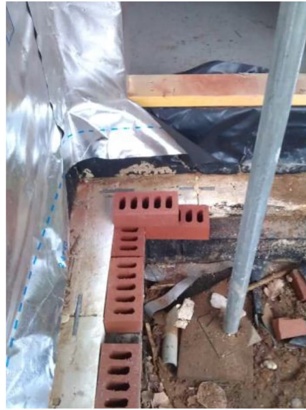
Figure 16: Brick outer leaf coming out of the ground alongside the insulated floor slab
