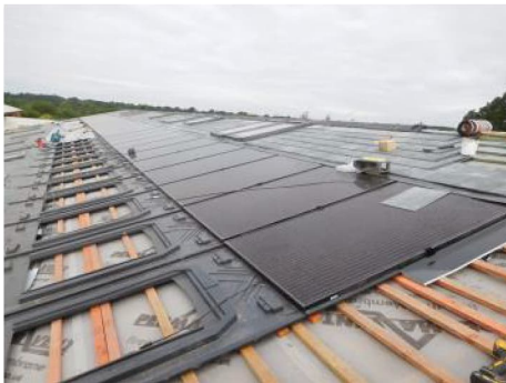
Figure 23: Slate roof with inline solar PV installation and rooflights
