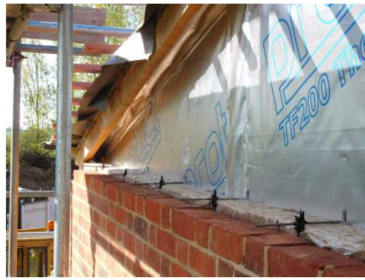
Figure 18: Brick outer leaf with insulated cavity under construction
