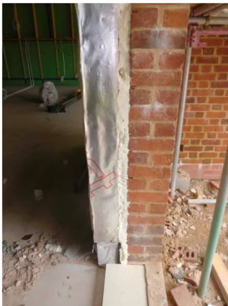
Figure 19: Insulated cavity closer
