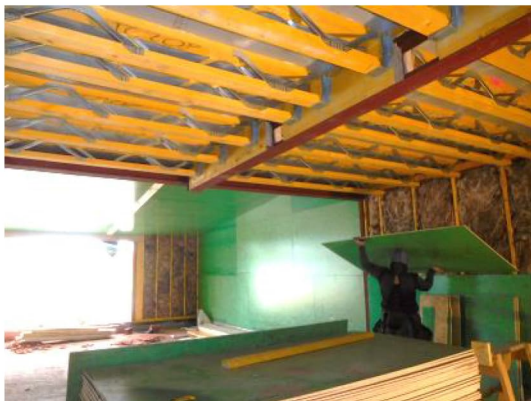
Figure 17: Propassiv airtight board being applied to insulated timber framed wall
