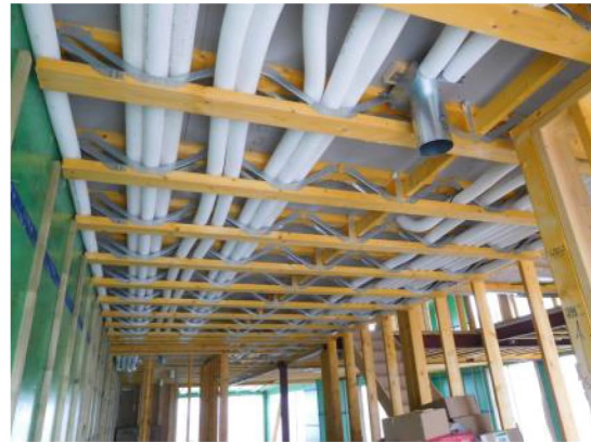
Figure 32: semi-flexible ventilation ductwork in intermediate floor void
