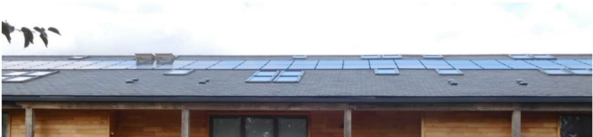
Figure 27: A 5.4 kWp solar PV system – inline roof installation
