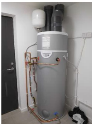
Figure 34: ASHP DHW cylinder
