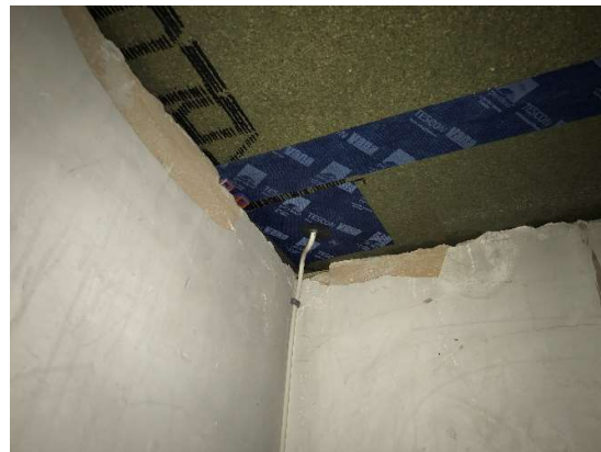
EPDM grommet in ceiling for single cable penetration
