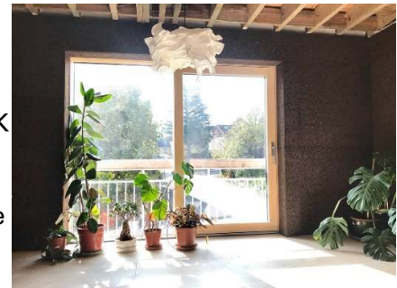
Tripple glazed Internorm sliding door and cork IWI on the reveals
