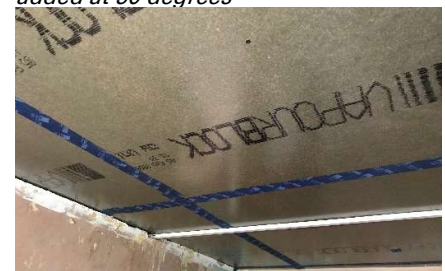
Vapour block board with taped joints
