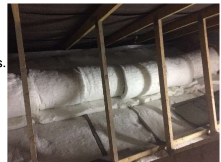
Installation of supaloft insulation between rafters with subsequent layers added at 90 degrees
