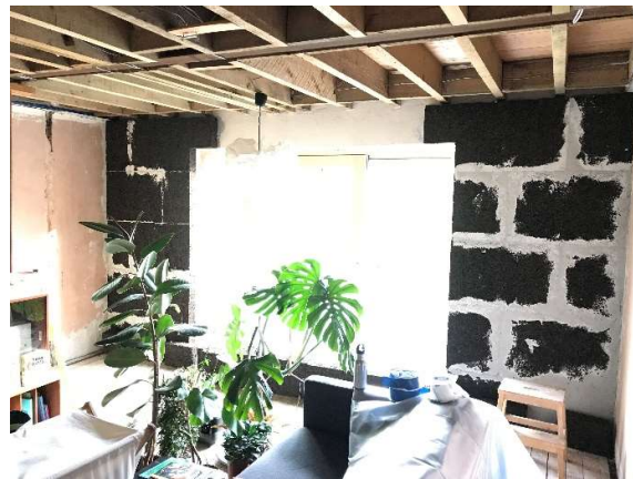
Cork Insulation being applied in living room.
