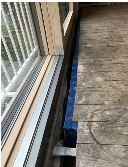
Airtightness of floor to front wall and sliding door: insertion of membrane and tape on outside face of joist with insulation between joist and brickwork
