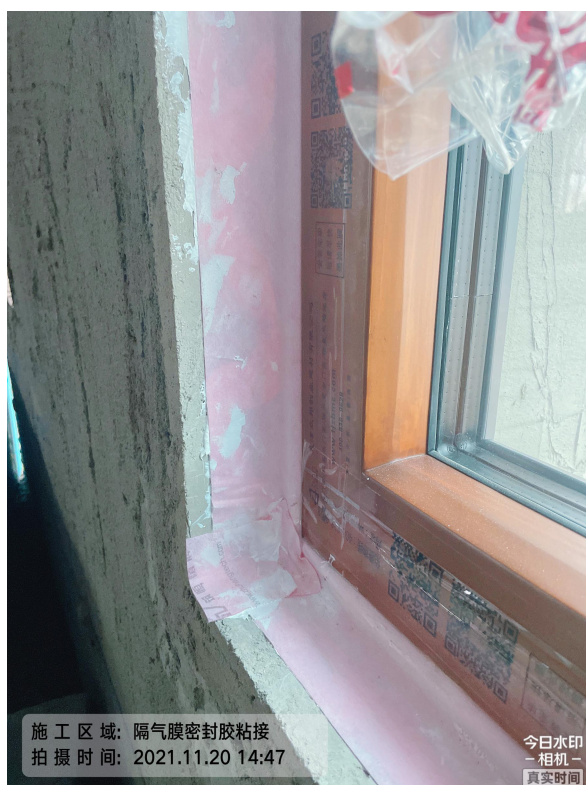
Construction of waterproof membrane and breathable membrane for external windows
