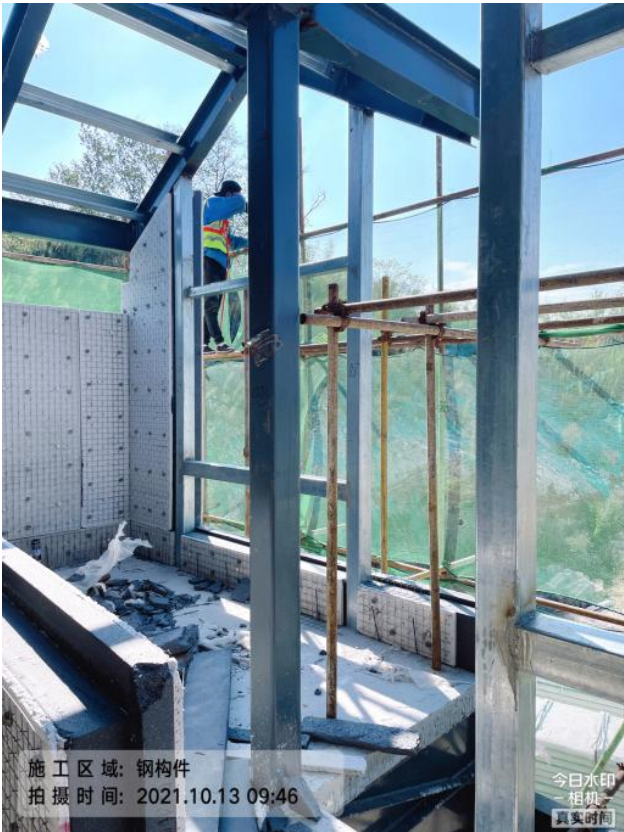
Assembled construction process of steel structure and exterior wall roof
