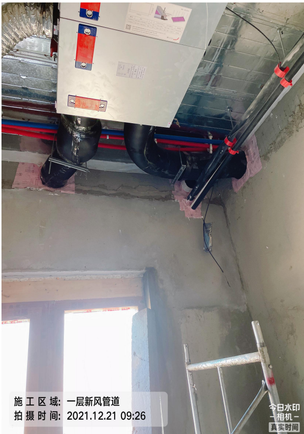
Fresh air duct on the first floor
