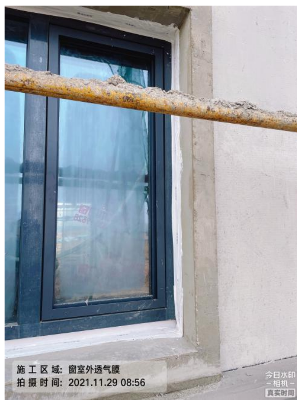
Construction of waterproof membrane and breathable membrane for external windows
