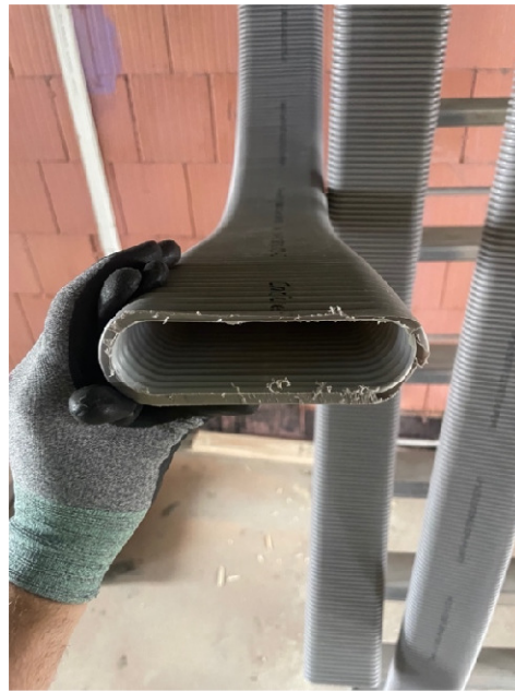
Manifold and ducts were installed within the ceiling zone between composite joists.
