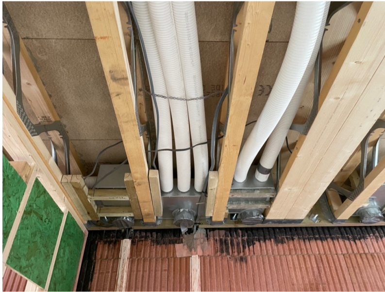
Manifold and ducts were installed within the ceiling zone between composite joists.
