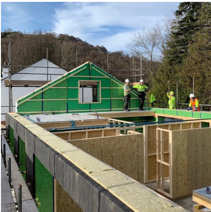
Installation of prefabricated first floor panels towards end of Day 1
