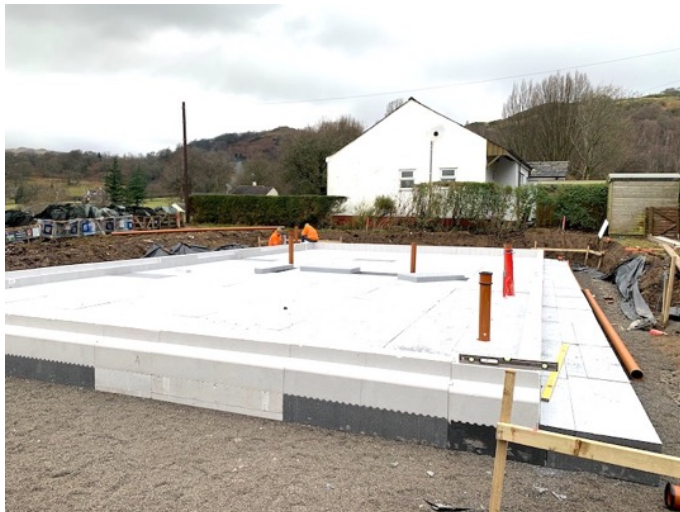
EPS insulation tray being installed
