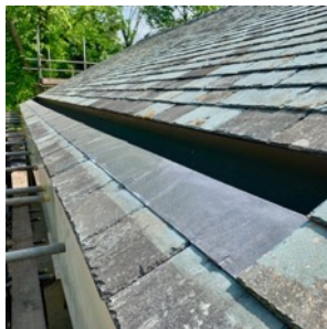
View of hidden gutter
