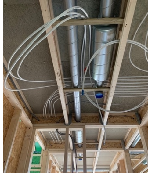
Ductwork and silencers located in first floor void
