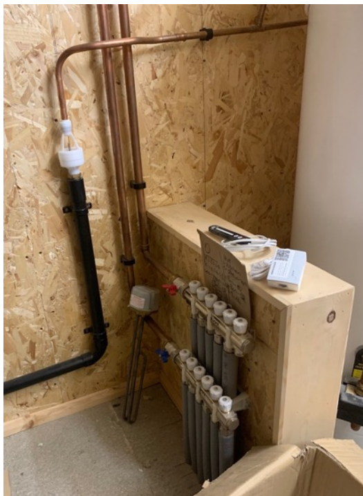
Hot water manifold system
