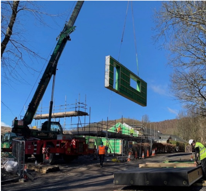
Prefabricated wall panels being craned into position
