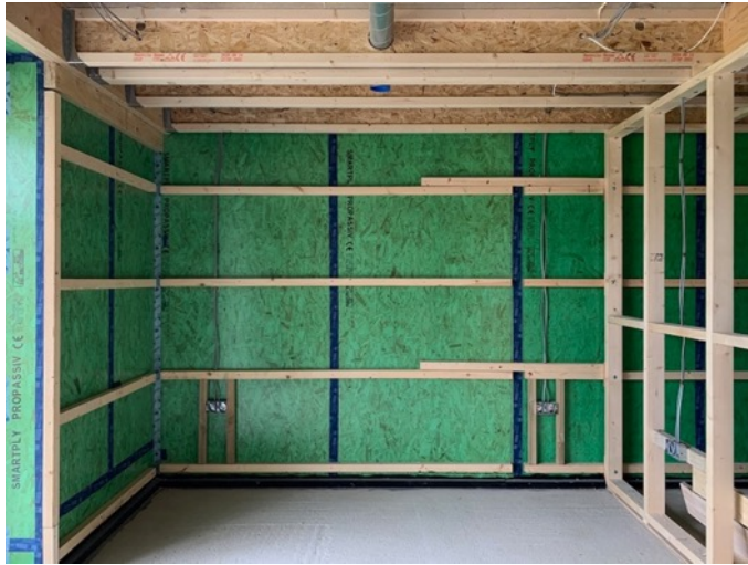
Construction view of prefabricated external wall and floor panels
