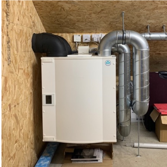
Systemair SAVE VTC 200R unit installed in plant room
