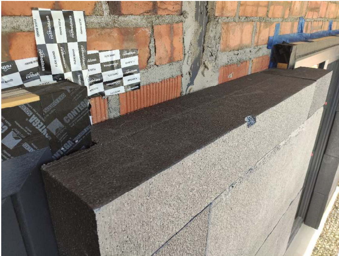
Facade insulation. Source: FERREIRA ARQUITECTOS
