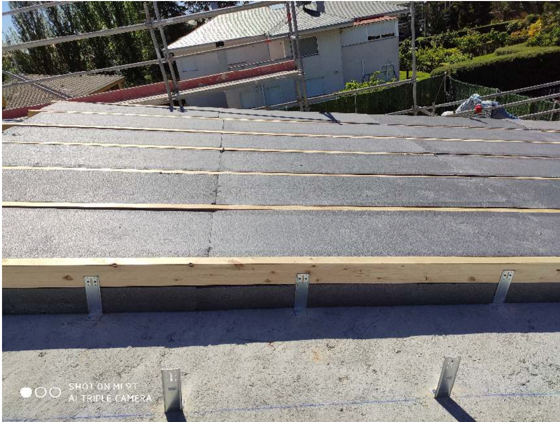
Roof insulation. Source: FERREIRA ARQUITECTOS
