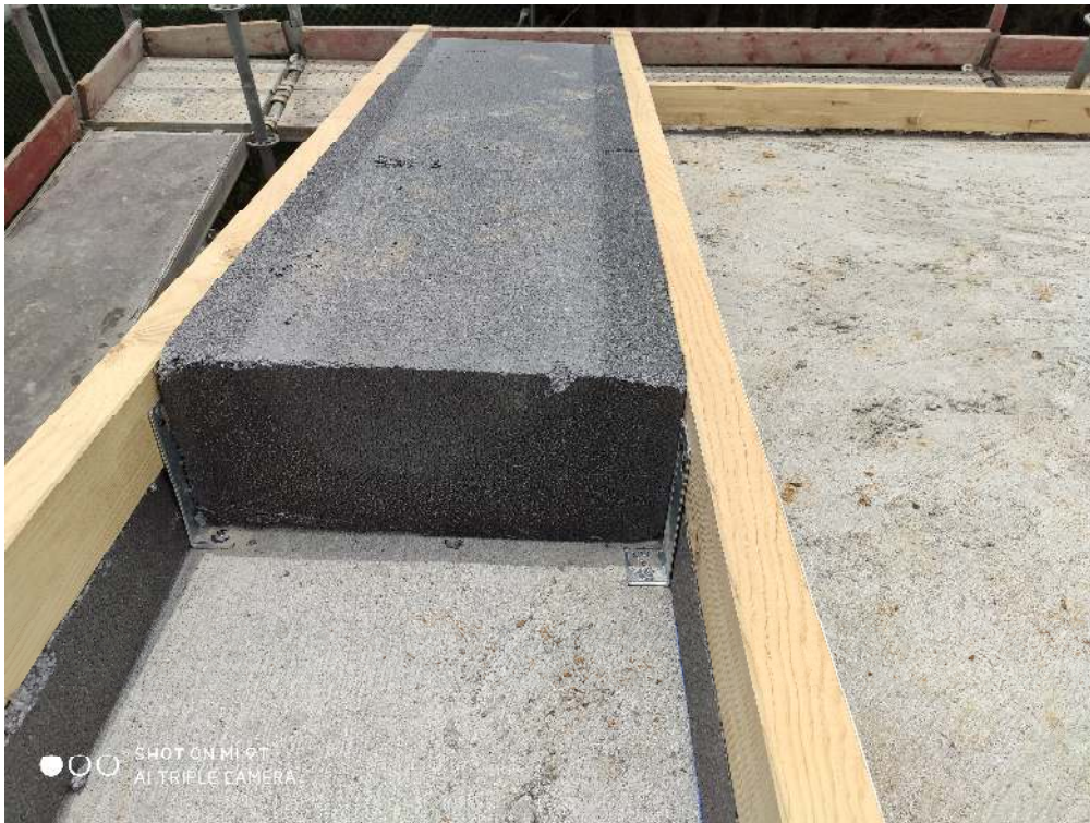
Roof insulation. Source: FERREIRA ARQUITECTOS
