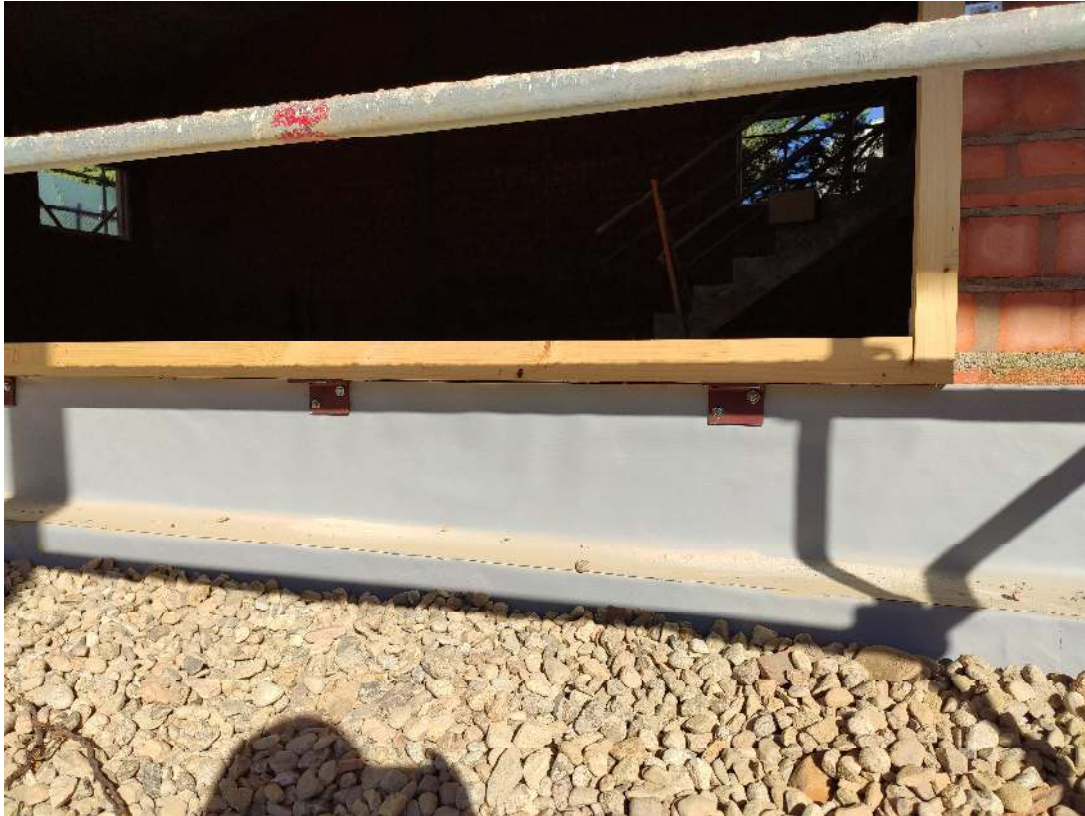
Window Instalation. Source: FERREIRA ARQUITECTOS
