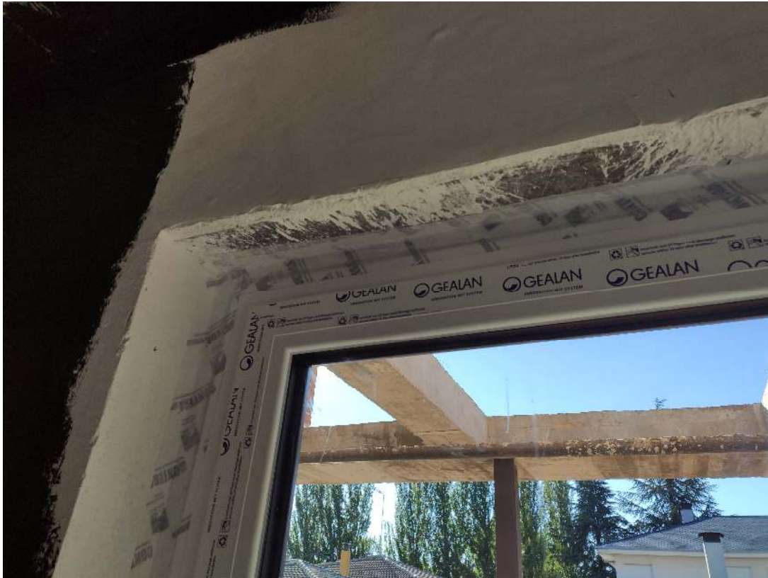
Window Instalation. Source: FERREIRA ARQUITECTOS
