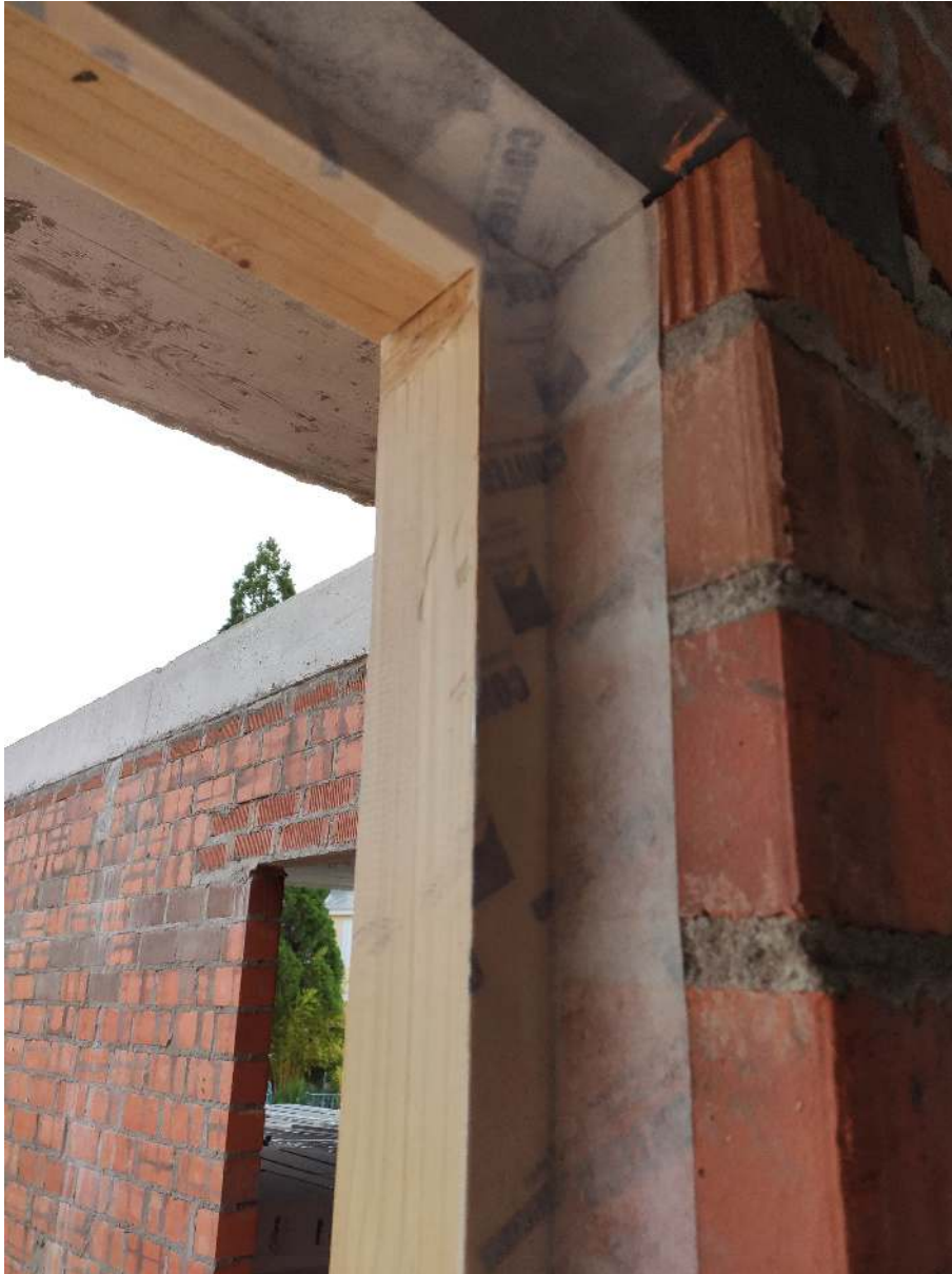
Window Instalation. Source: FERREIRA ARQUITECTOS
