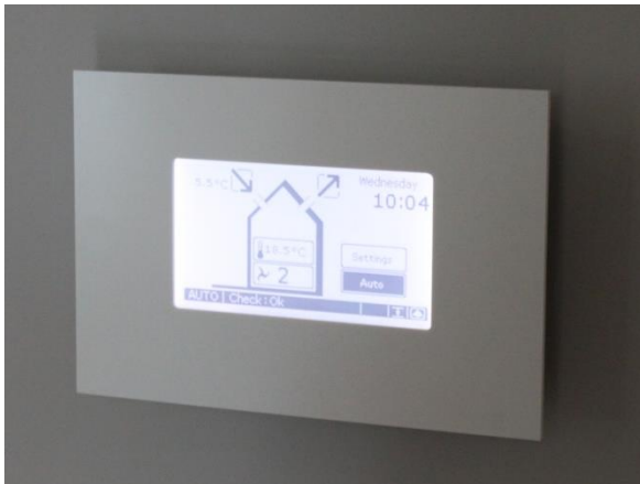
Ventilation control unit located in dining room
