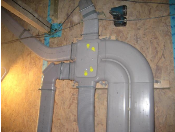
Supply and extract manifolds
