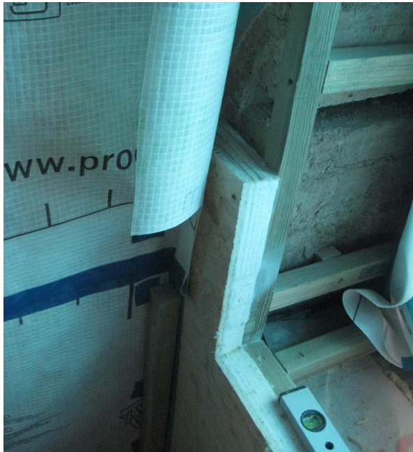
Wall type C: Aerogel insulation wall lining
