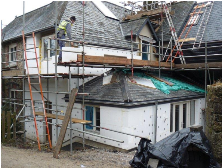
Wall type D: showing installation of EIFS
