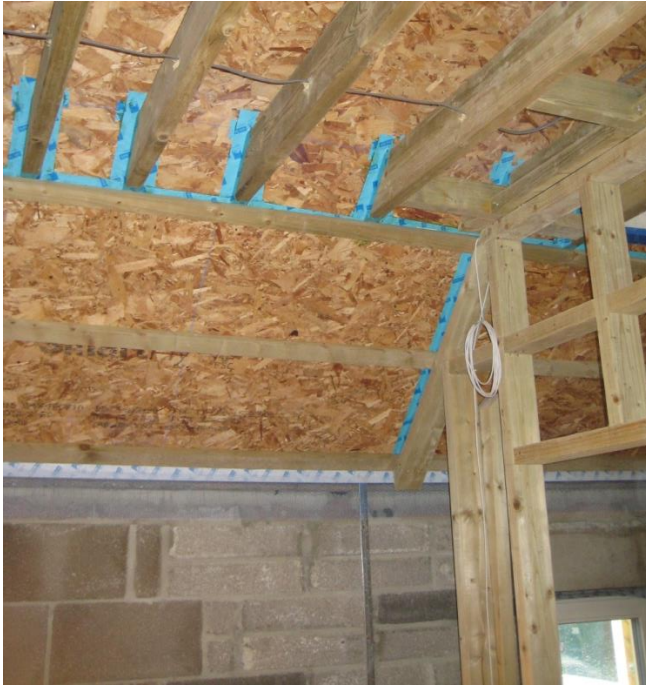
Air barrier to new extension: the air barrier in the roof was formed by OSB and linked to the plastered wall with a plaster tape.
