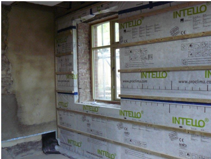
Wall type A: showing VCL and service void
