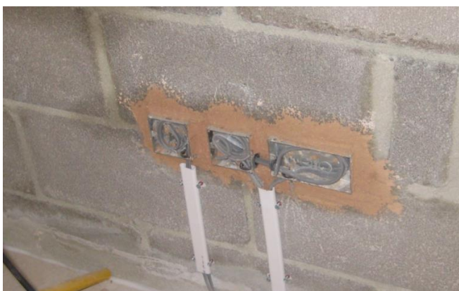
Air barrier to new extension: Sockets were fully bedded into mortar and trunking cut short to allow for continuous plaster layer (air barrier).
