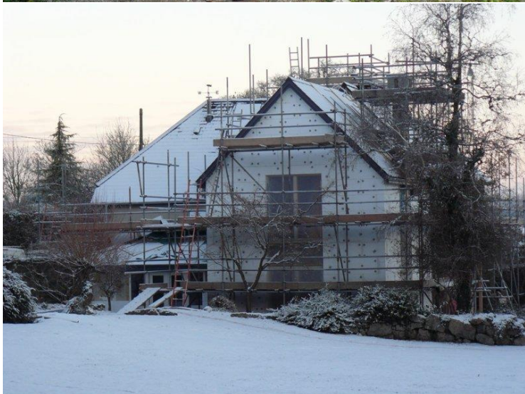
Wall type E/F: showing installation of EIFS
