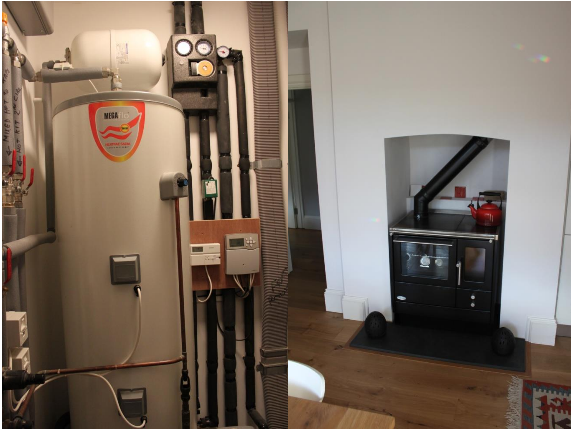
Thermal store and air tight range cooker with backboiler option replicating a traditional feature.
