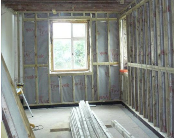
Wall type A: showing foamglass warm foot detail
