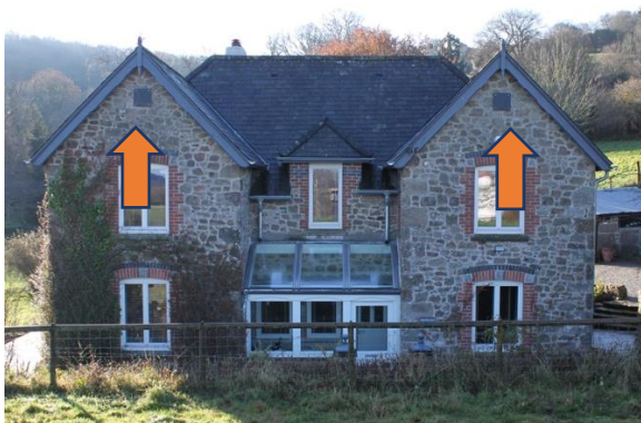
MVHR intake and exhaust behind slate louvres on north facing gables
