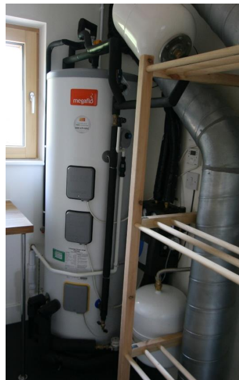
30 Baxi evaluated solar hot water tubes on roof, feeding 210 litre Megaflow hot water cylinder.
