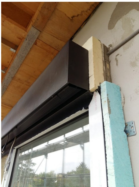
Details of the raffstore and the insulation behind the box
