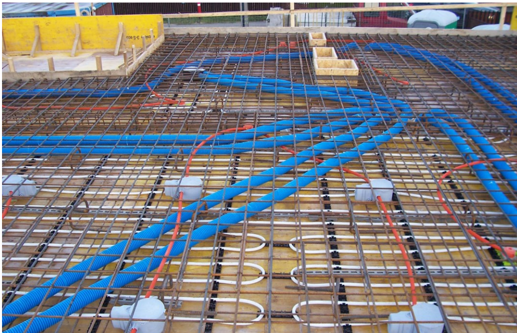
Ventilation pipes
