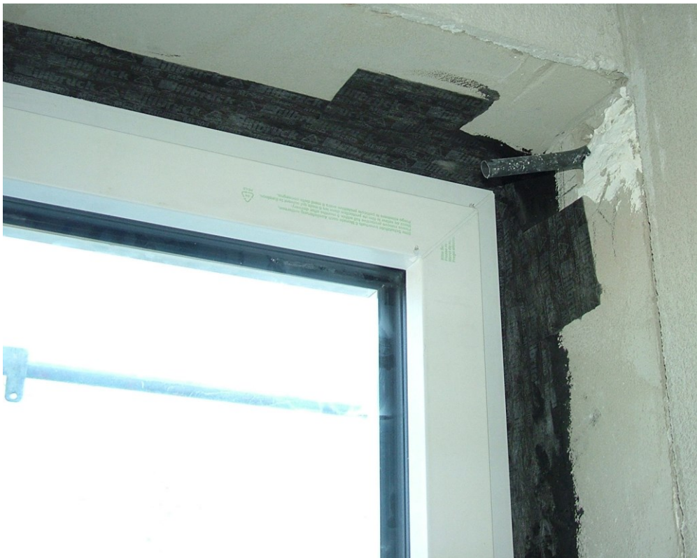
flexible window membrane glued on the plaster
