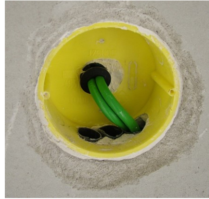
Dörken Delta-Reflex vapour barrier and Kaiser airtight rubber sealing plug.
