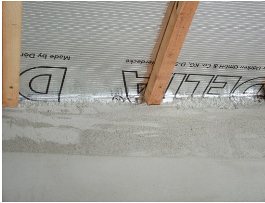
Dörken Delta-Reflex vapour barrier and Kaiser airtight rubber sealing plug.
