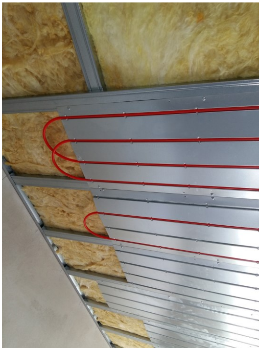
In First Floor, the pipes for the ceiling heating (and cooling) were built into the plasterboard ceiling.
