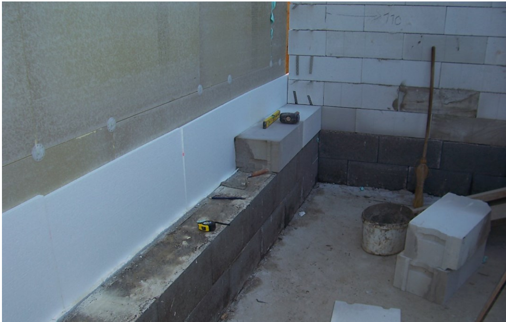
240mm PIR Insulation between the garage and the thermal envelope.
