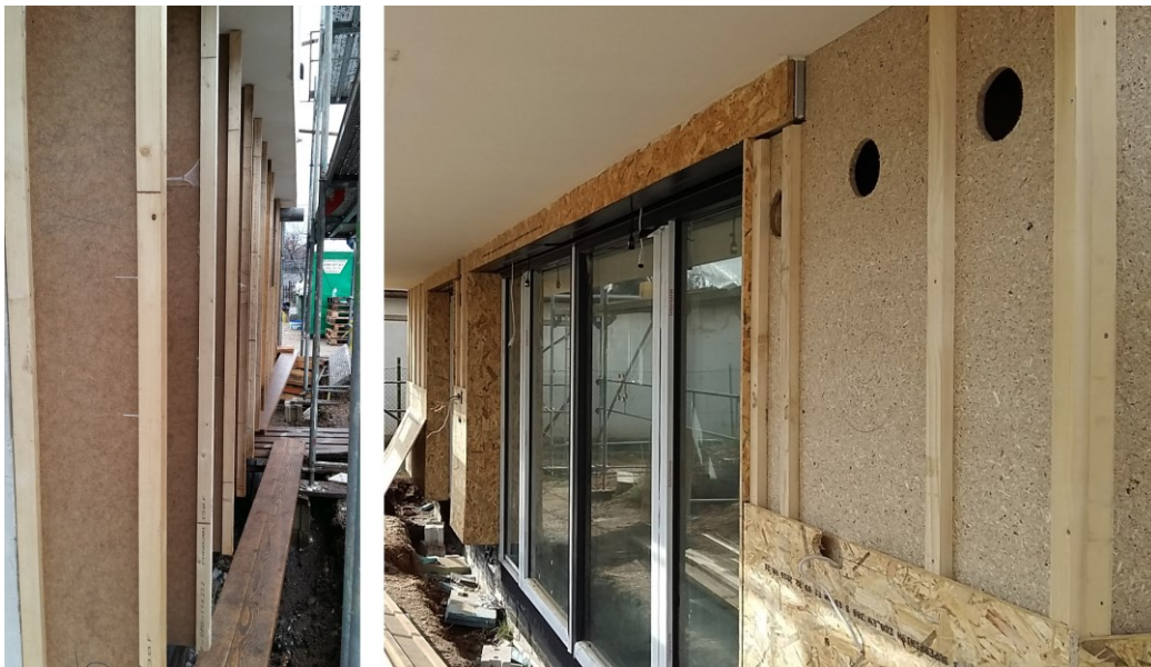
Ground floor external wall insulation
