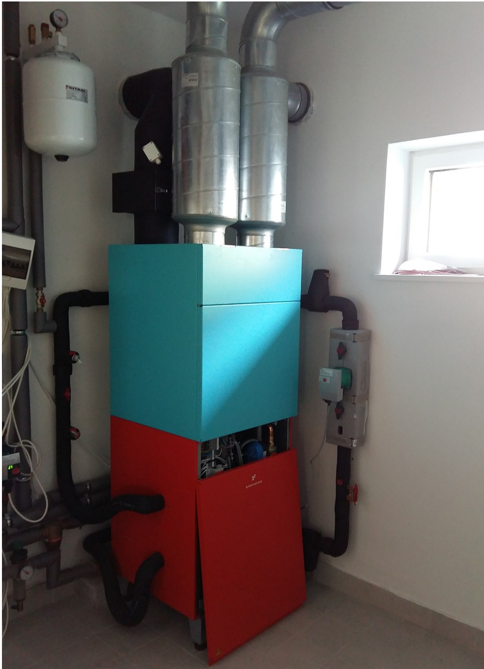
Drexel & Weiss X2 S5 compact heat pump unit
