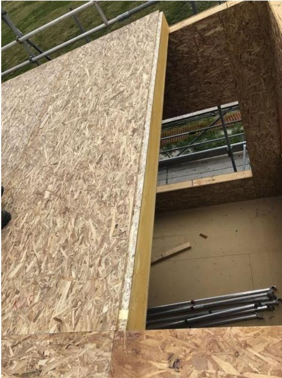
Roof panel installation
