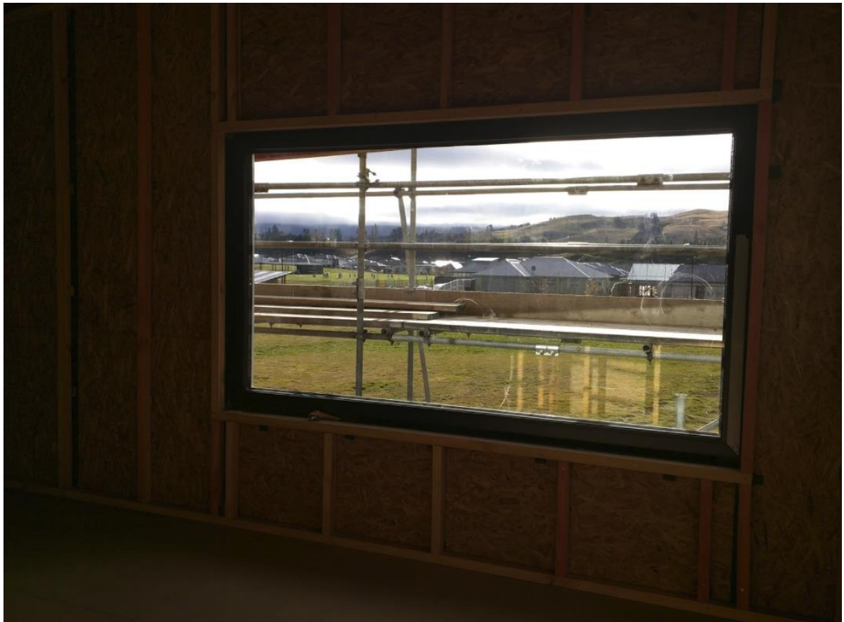
Installed window, prior to installation of internal insulation and linings. OSB airtightness layer.
