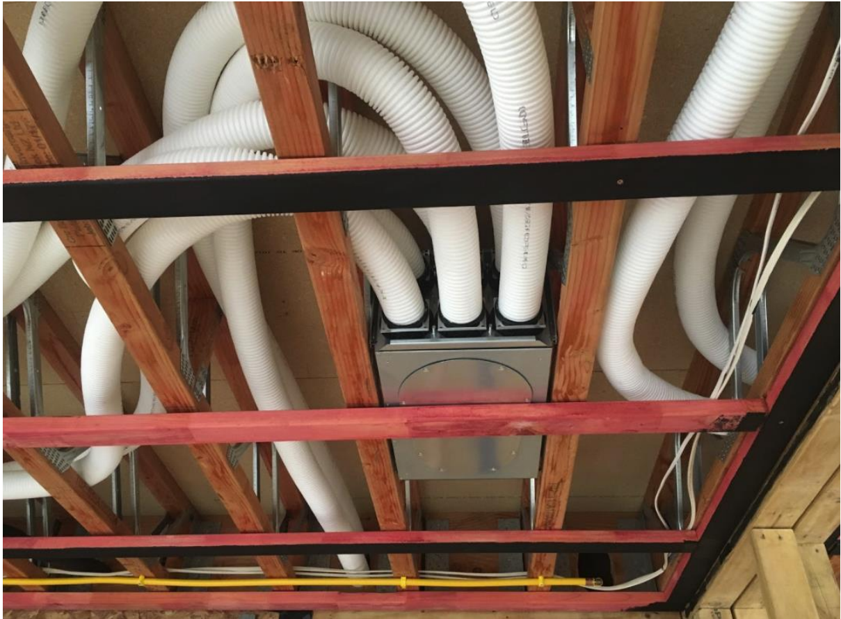
4. Supply air manifold between joist in intermediate floor.
