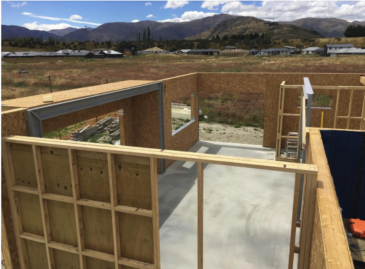
Ground floor SIP panels in place
