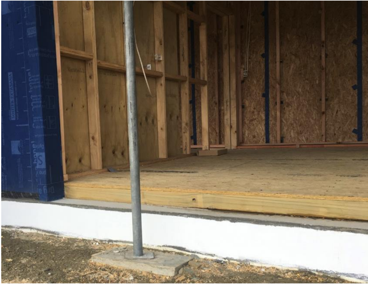
Edge of overlay insulation build up visible prior to installation of doors
