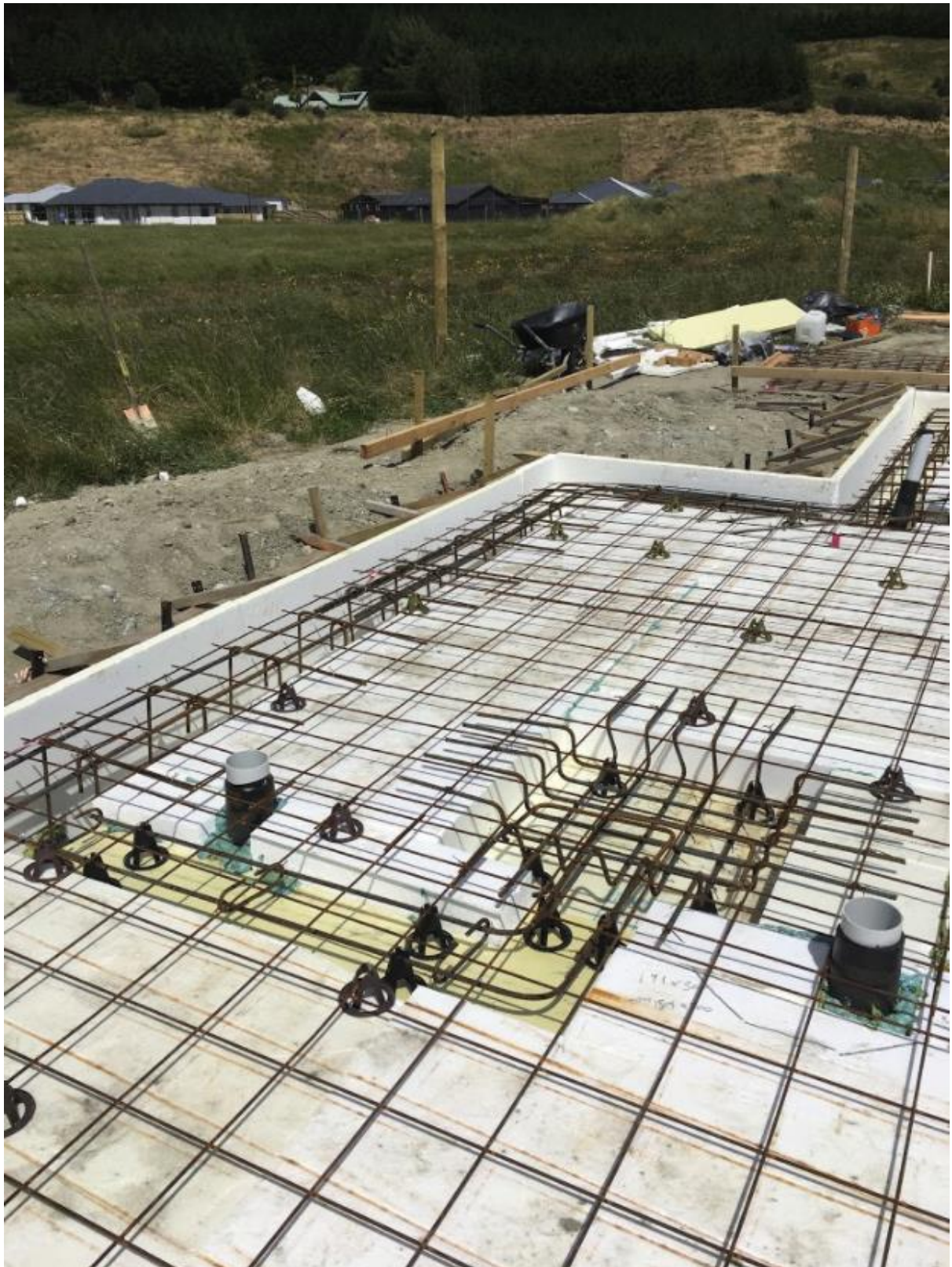
Under slab and perimeter insulation, prior to concrete pouring.
