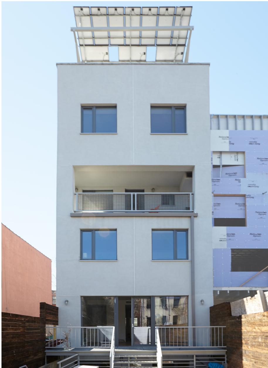
North (Rear) Facade
