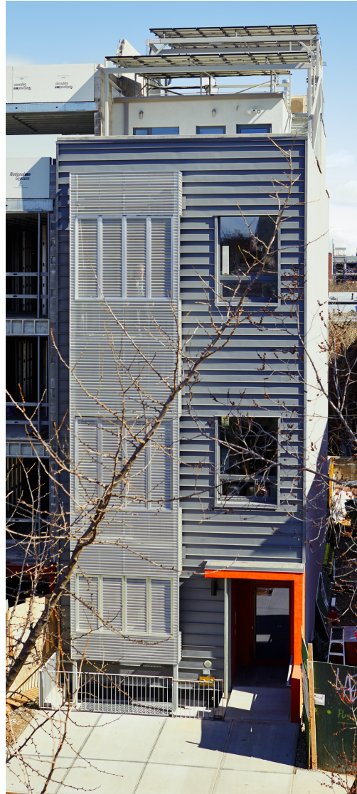
South and angled view of East Facade (NOTE: Adjacent Building at West Facade)
