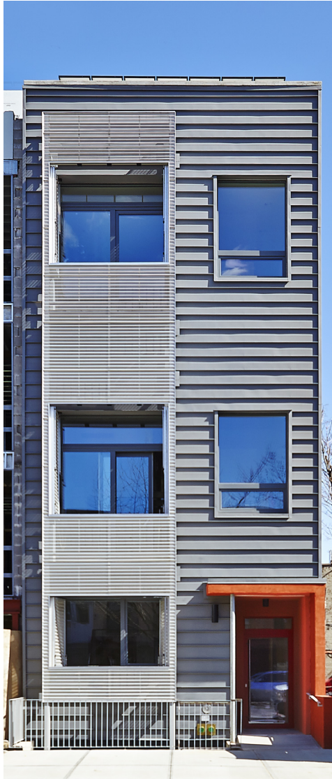
South (Front) Facade
