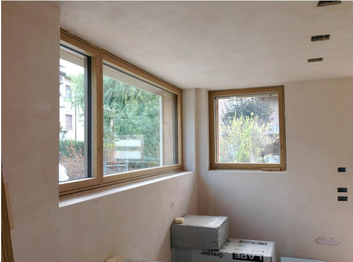
Windows installed in the living area.
