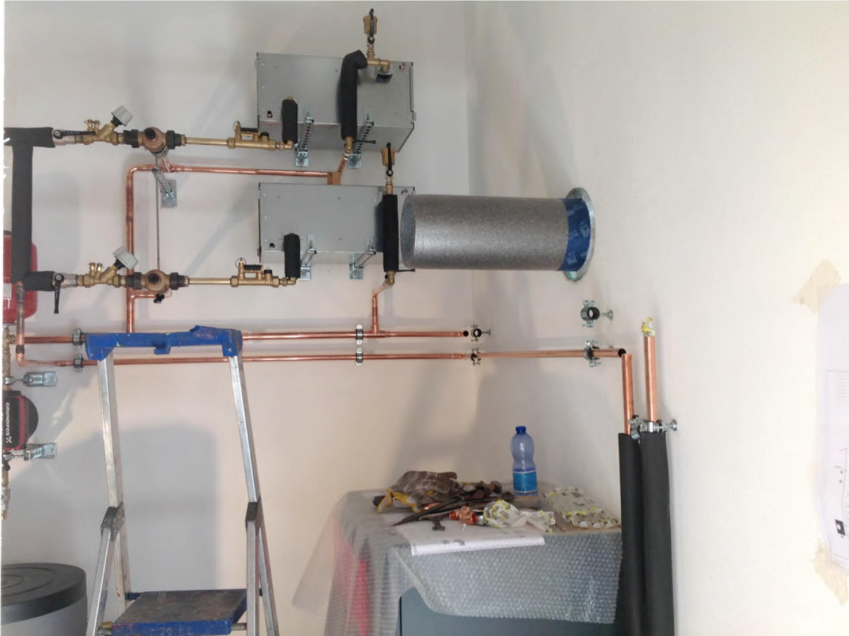
Heating system being installed in the mechanical room.
