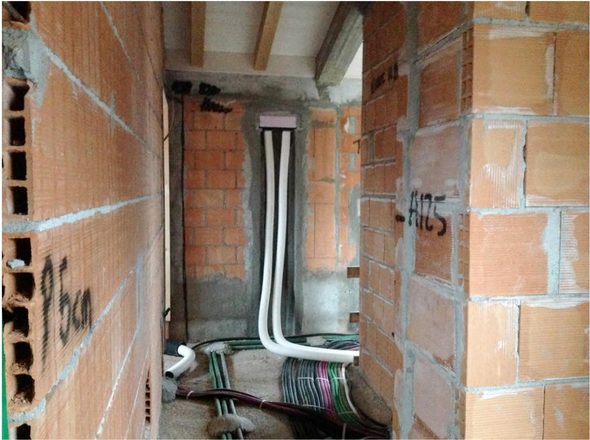
Installation of Extract Air ductwork in future laundry room.
