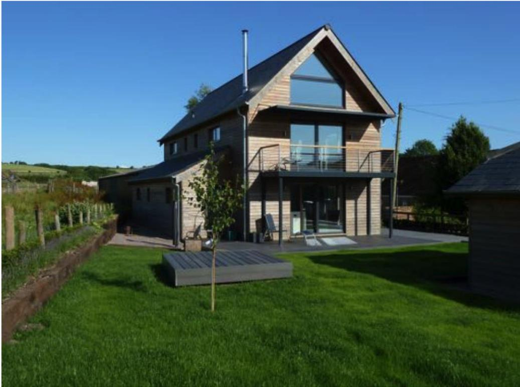
West view: showing solar shading. Decking in foreground covers aeration sewage treatment plant.
