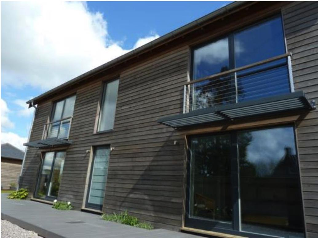
**South elevation:** main entrance door in centre. Sliding doors to main rooms and fixed window to stairwell above entrance. Fixed solar shading over ground floor windows. Deep roof overhang.
