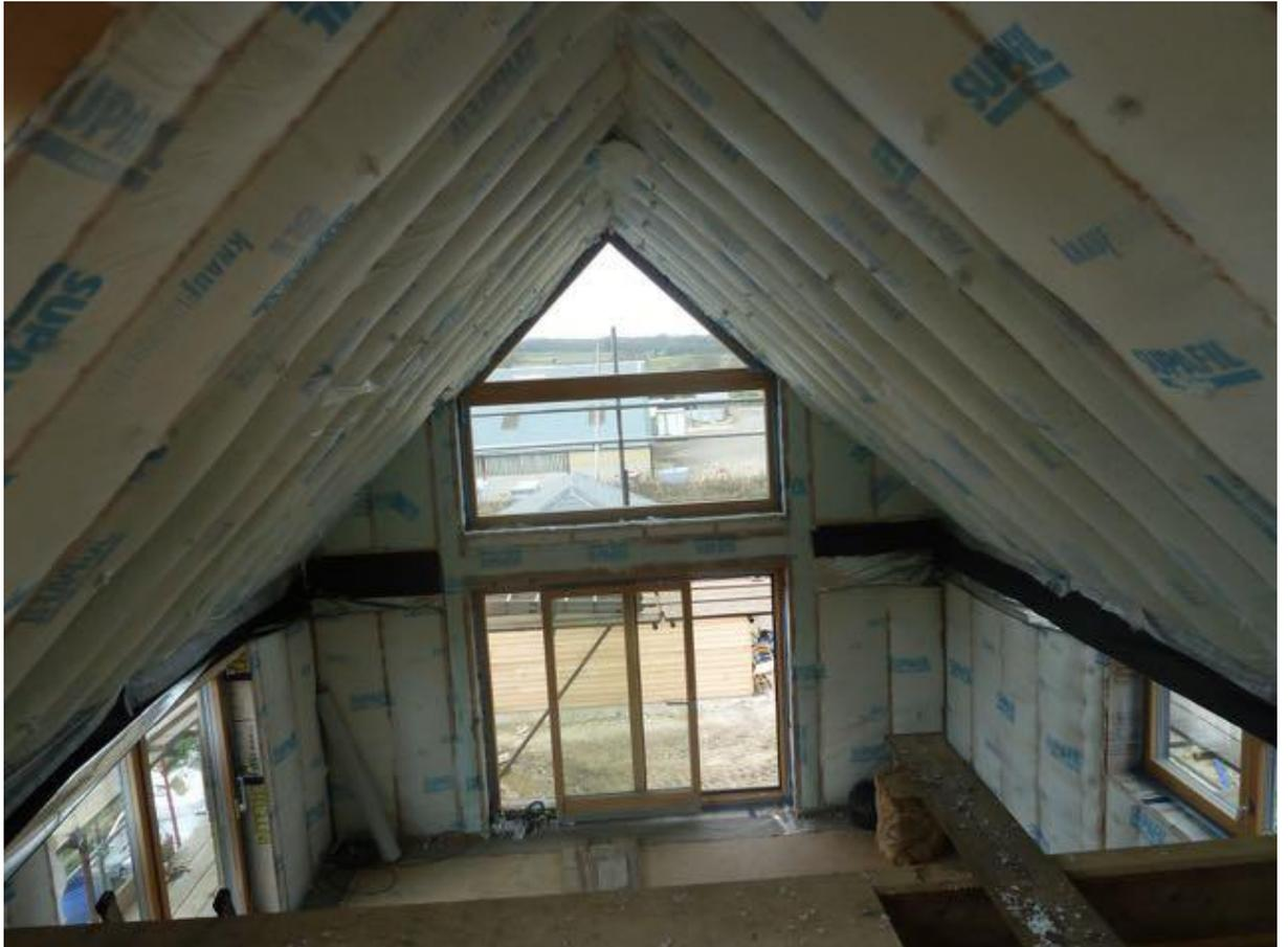
5.2.3 I was keen to avoid any steelwork in the structure so as to avoid cold bridges. Unfortunately the timber frame fabricator and their engineers were fairly traditional and would not entertain designing entirely without steel. A portal frame was required to the large west facing windows, but all other steel omitted. To mitigate the impact of the steelwork, I ensured that the steel was placed as close to the inside face as possible, with high performance insulation wrapped around it.
