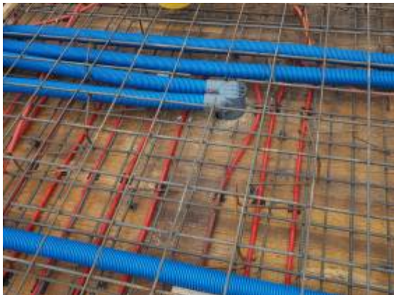
Ventilation ducts installed in concrete slab.
