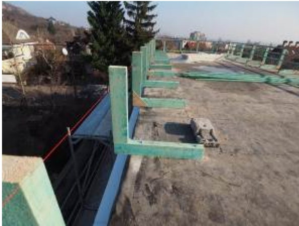
Construct of the roof attic, and isolating the roof slab (Reinforced concrete slab, vapor barrier foil, isolation, concrete slope, waterproofing, green roof)
