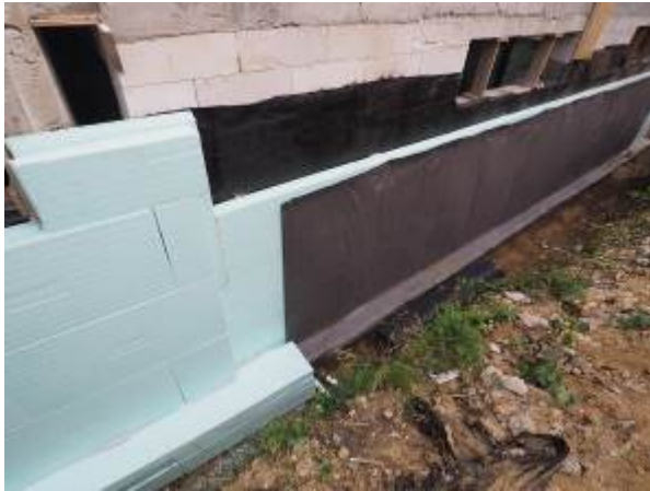
Isolation under ground (Reinforced concrete wall with Expert EPS isolation - thickness is various 15, 25 cm)
