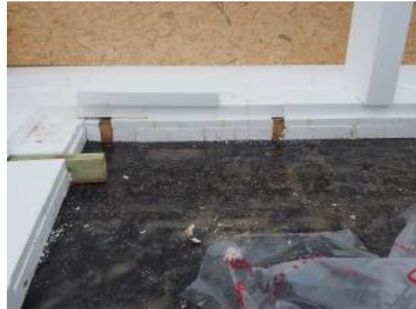
Construct of the roof attic, and isolating the roof slab (Reinforced concrete slab, vapor barrier foil, isolation, concrete slope, waterproofing, green roof)
