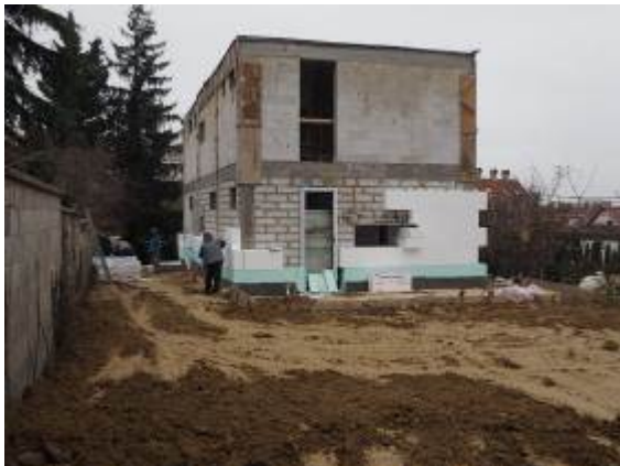
Constructing the exterior walls (The exterior walls made of autoclaved concrete elements (Ytong) with reinforced concrete pillars and 25 cm external EPS isolation)
