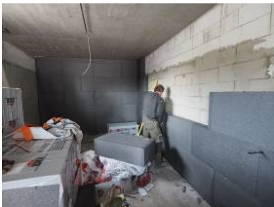
Constructing the basement interior wall between the heated zone and the garage (Ytong walls with 15 cm external graphitic EPS isolation)
