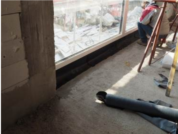
Making airtight joint between concrete slab and glass structure using bituminous foil.
