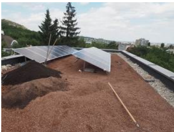
Making the ground for green-roof
