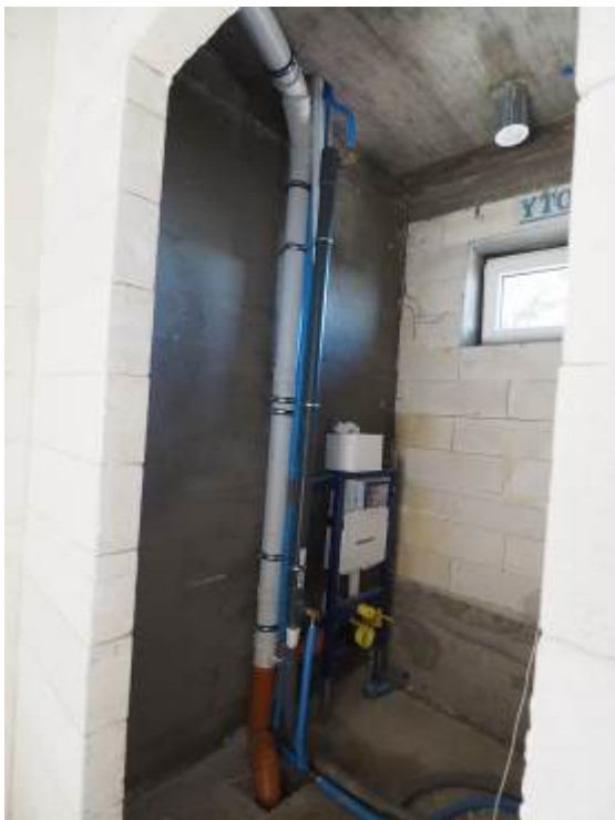
Internal smoothing made behind inbuilt technical equipment
