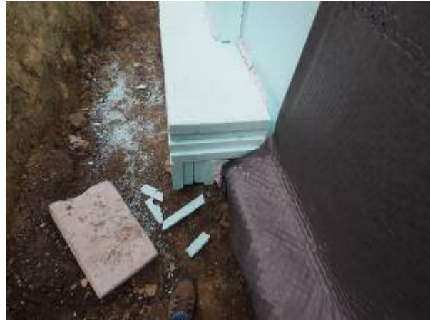
Isolation under ground (Reinforced concrete wall with Expert EPS isolation - thickness is various 15, 25 cm)
